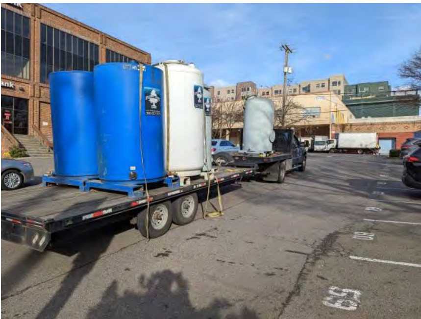
Photograph 8. Vapor GAC Removal (March 2022)
