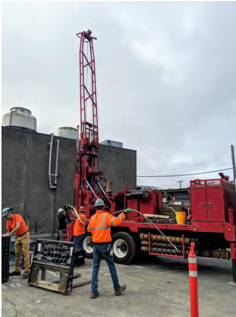
Photograph 1. Electrode Installation in KeyBank Parking Lot (2019)
