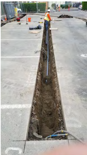
Photograph 2. Electrode Row D Trench (2019)
