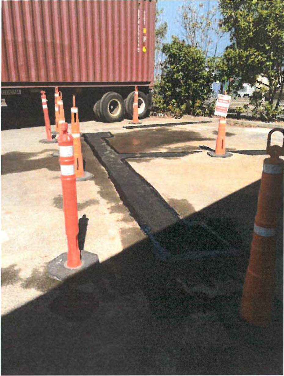
Traffic rated trench completion in warehouse parking lot.
