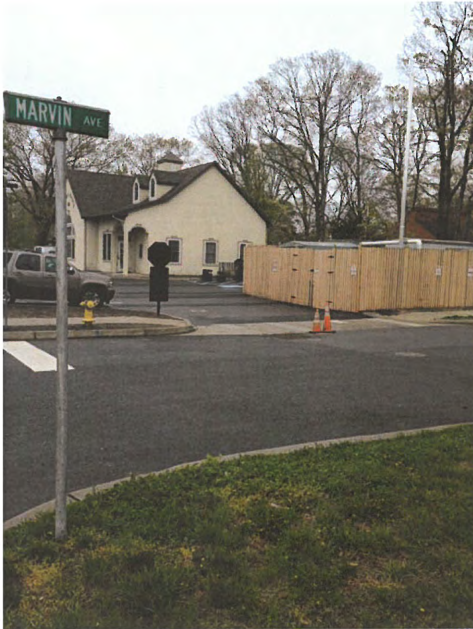
Small equipment compound with privacy slat fence. Note stack from carbon vessels rising above the compound.
