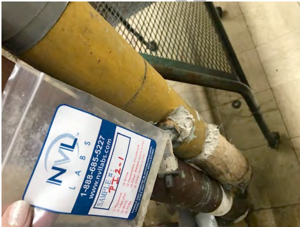
Photograph 4 – Pipe Insulation (PI2-1), Production Building
