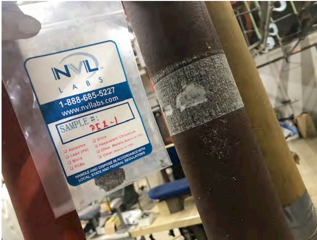
Photograph 3 – Pipe Insulation (PI1-1) Production Building
