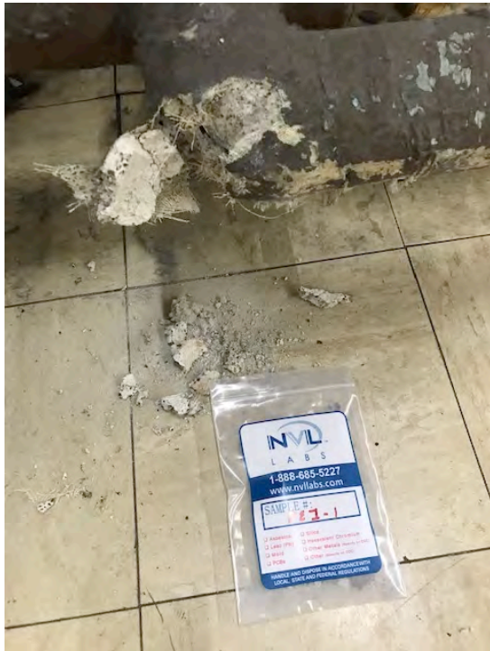
Photograph 1 – Pipe Elbow (PE1-1), Production Building
