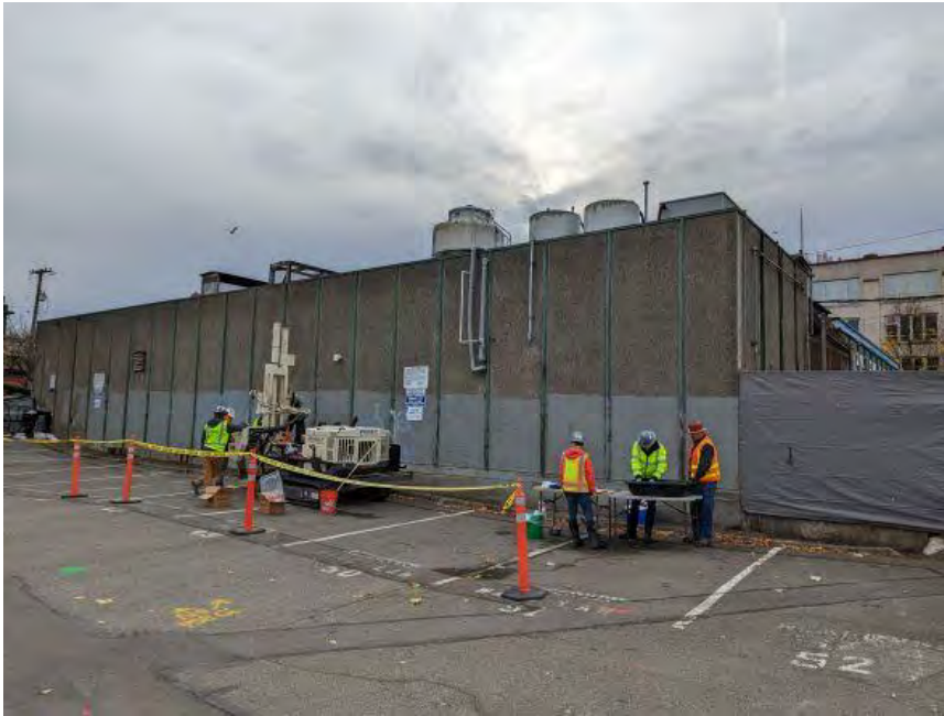
Photograph 5. Confirmation Soil Borings (November 2021)
