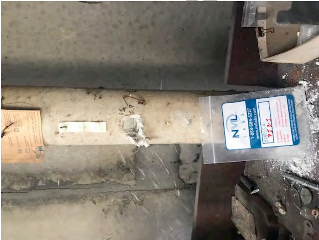
Photograph 6 – Pipe Insulation (PI1-3), Maintenance Building
