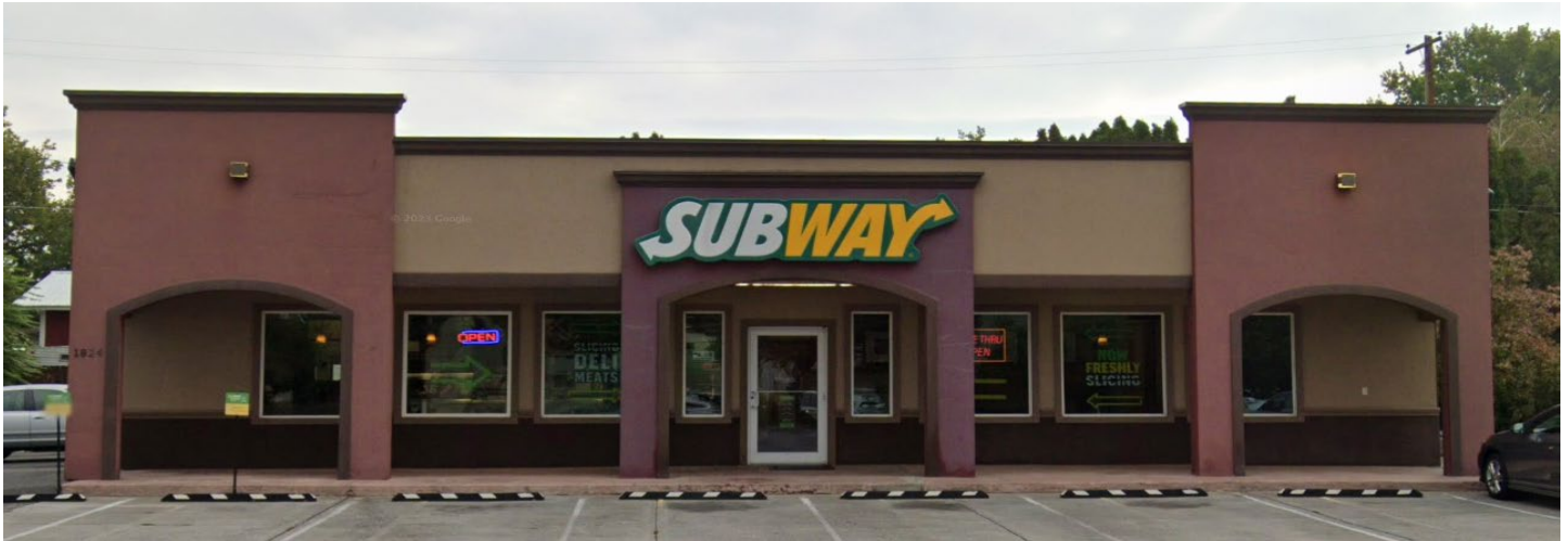
Former 7 Eleven 25821 – Photo courtesy of Google Street View
