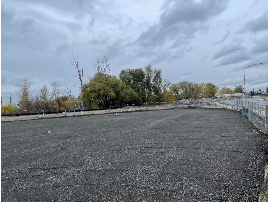
Photograph 1. View of proposed Building 2A footprint with building footprint excavation backfilled and stormwater cover placed and compacted. Looking northeast.
