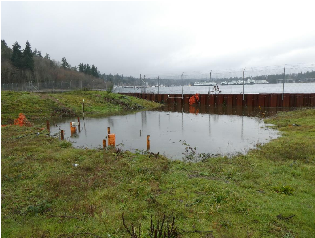
Western sheet pile wall and extraction wells with standing water
