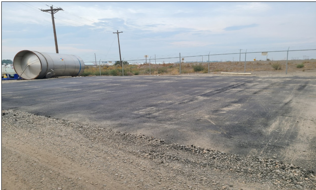
Former wash pad near the north east corner of the property
