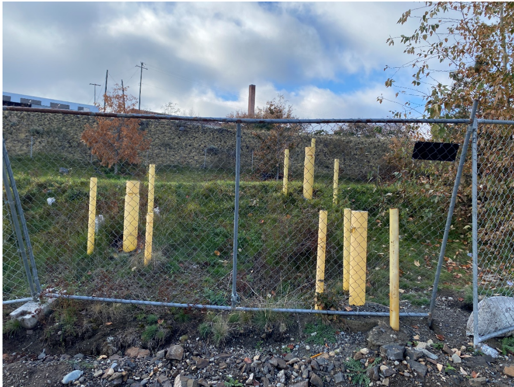
1. View of monitoring well cluster MW8 and compromised perimeter fence (right side) on the former SGP property (looking southwest).
