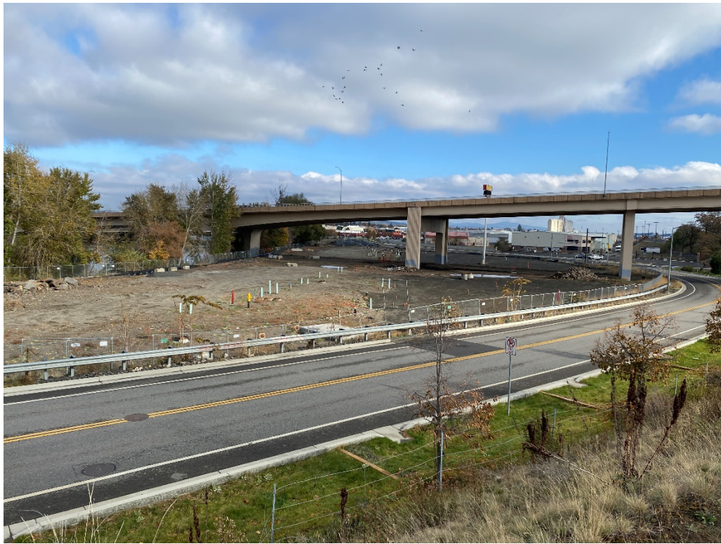
1. View of former SGP portion of the site (looking northeast).
