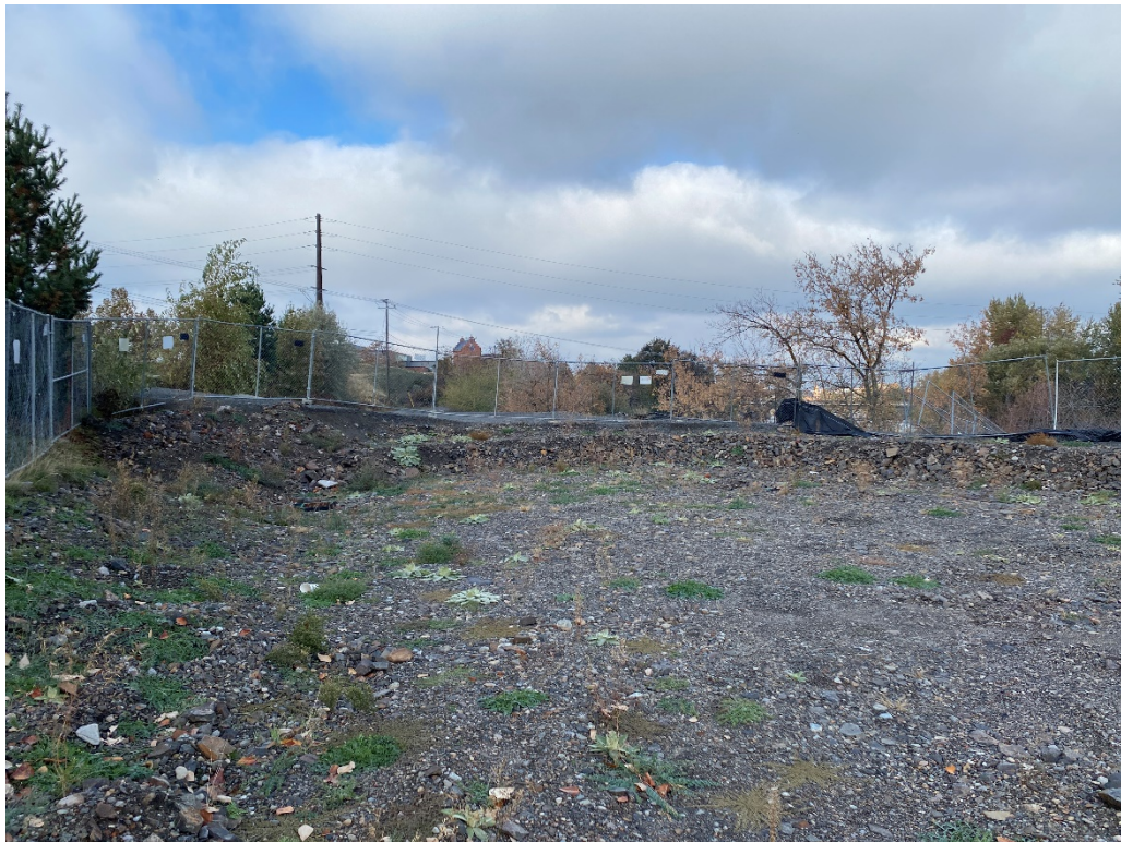
2. View of the new west infiltration gallery (looking west).
