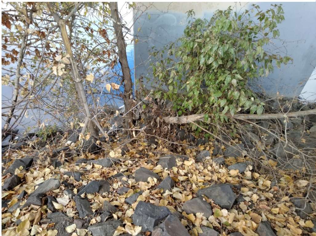
2. View of cleanup action shoreline armoring transition zone with cut down tree on the former SGP property (looking north).
