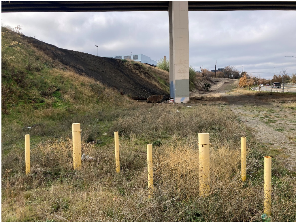
2. View of ATC portion of the site and ATC monitoring wells (looking west).
