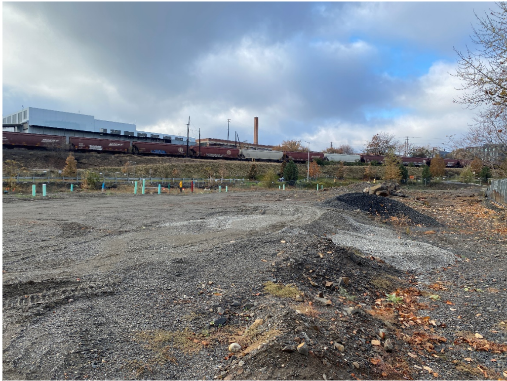
1. View of the elevated area of soil observed in the western portion of the former SGP property (looking southwest).
