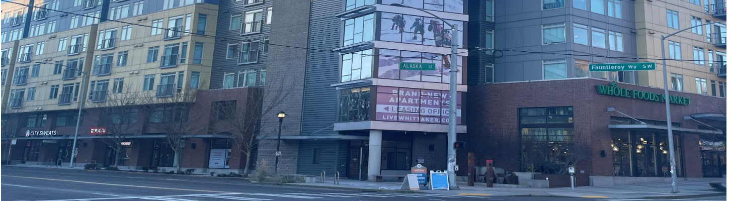
SKS Shell Station cleanup site today.
