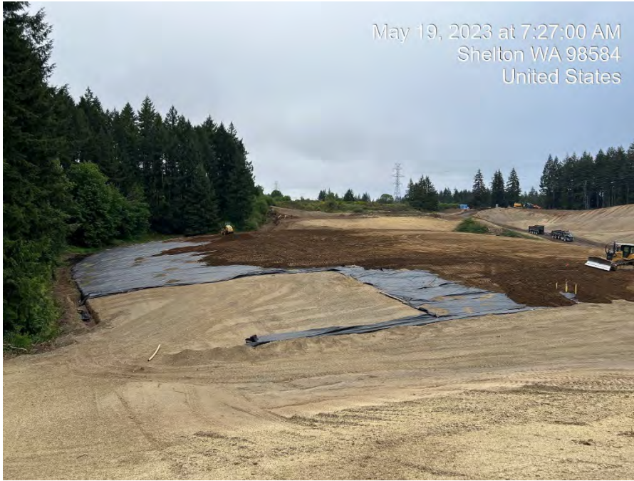
Photograph 7. Installation of geotextile barrier. Photo faces north-northeast.
