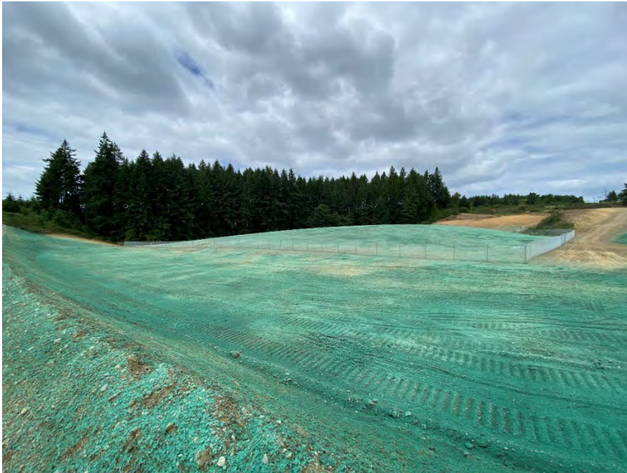
Photograph 9. Hydroseeded areas following completion of cleanup construction. Photo faces northwest.
