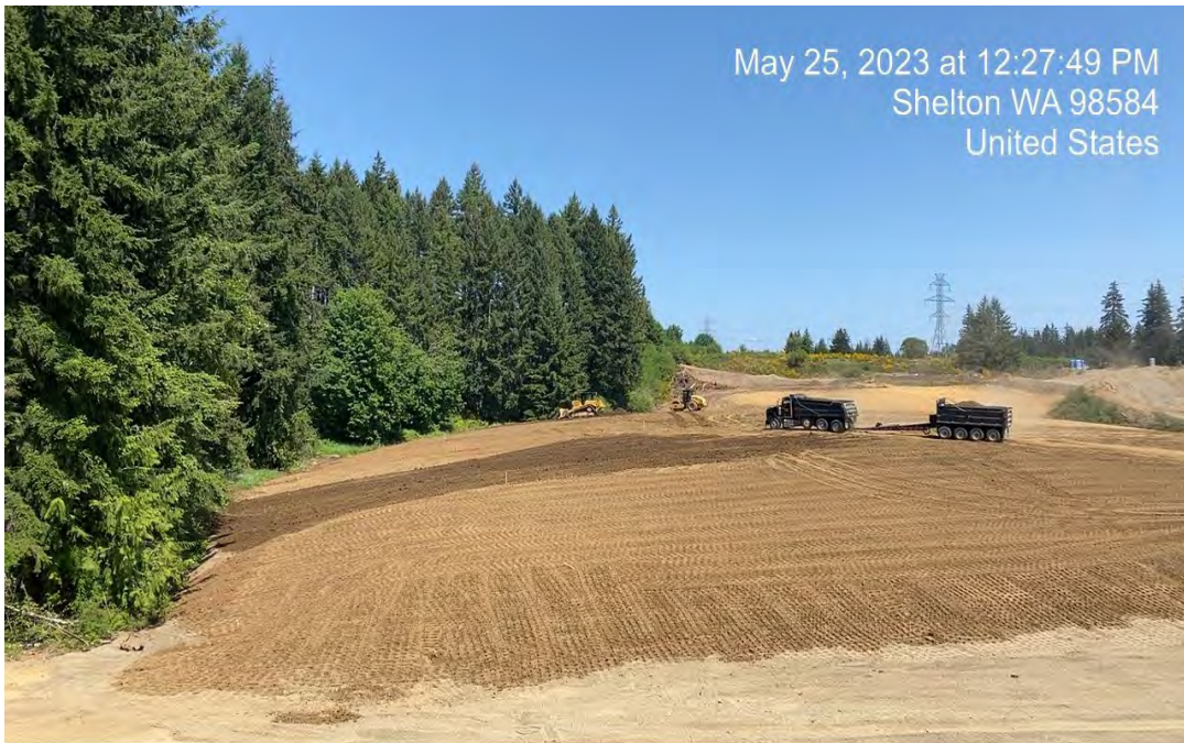
Photograph 8. Placement of low permeability soil overlying geotextile barrier. Photo faces north-northeast.
