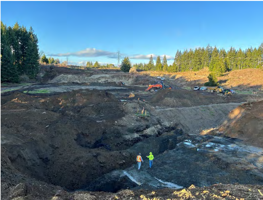
Photograph 4. Landfill waste relocation excavation on south-adjointing property. Landfill waste shown in dark-colored layers. Photo faces north.
