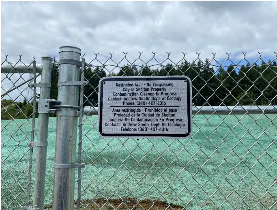
Photograph 11. Typical fencing and signage installed around soil cap on the Property.
