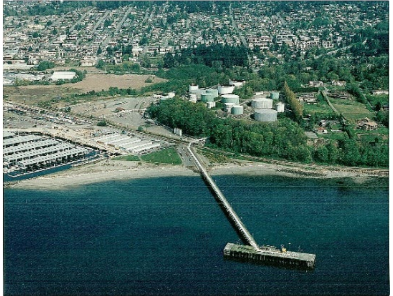
Historic view of fuel terminal
