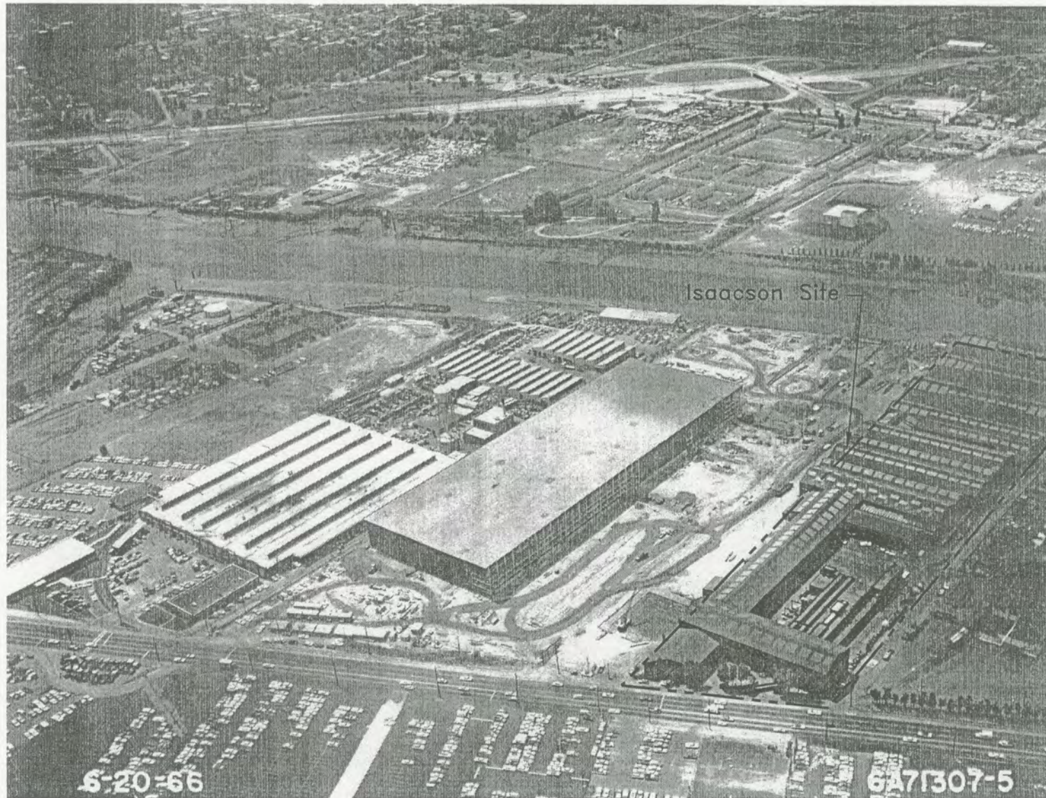
View to Southwest
