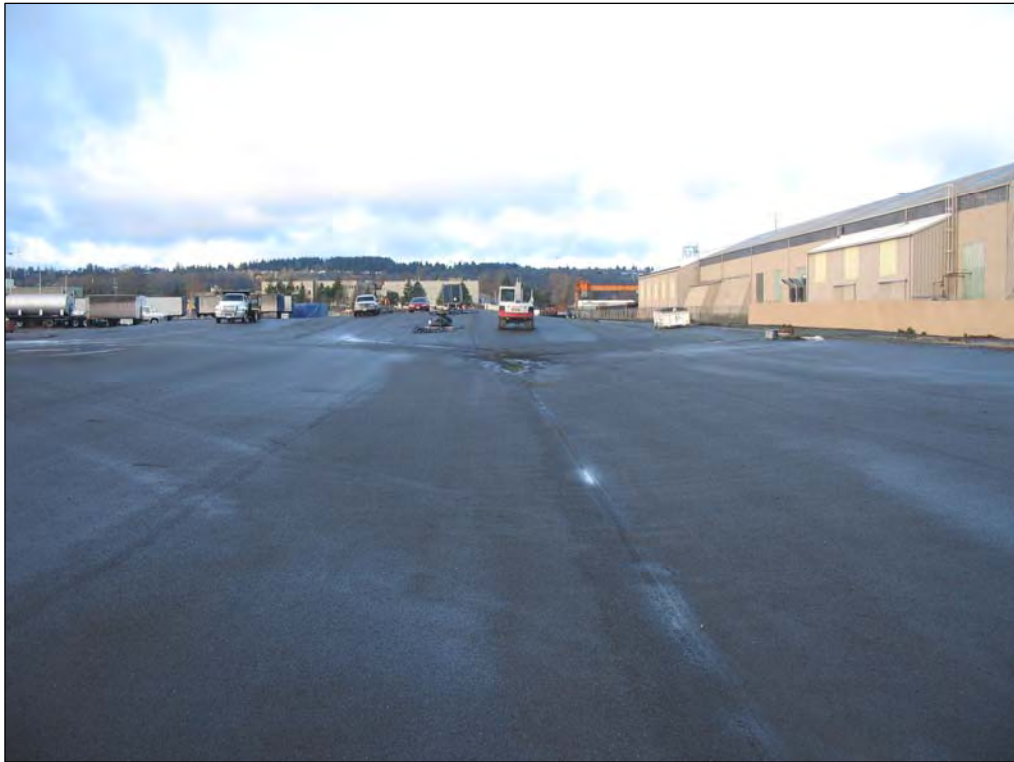
2. Looking west from near the eastern boundary of the subject property.
