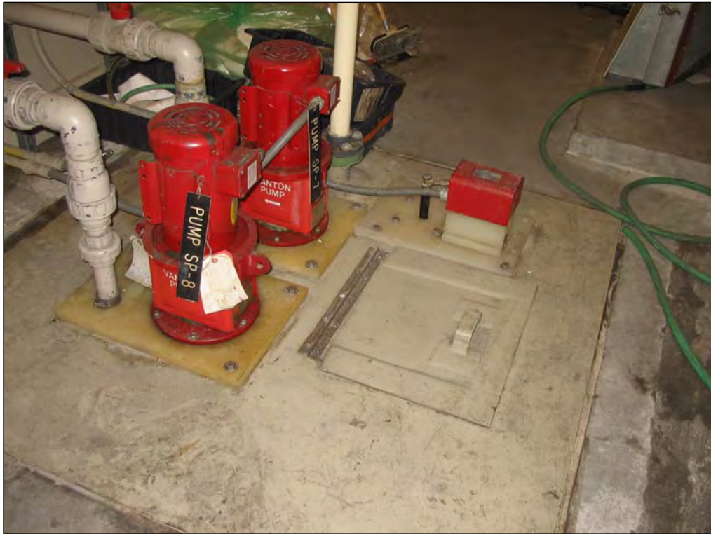
6. Former brush plating sump located in the southwestern portion of Building 14-01.
