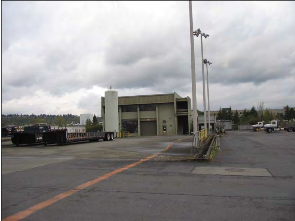
9. Former hydraulic systems test pad.
