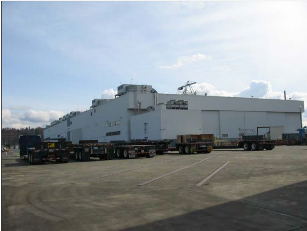
10. Looking southeast at Buildings 14-14 and 14-01.
