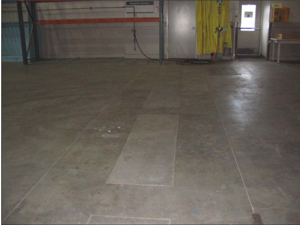
5. Former (patched) wastewater trenches in the southwestern portion of Building 14-01.
