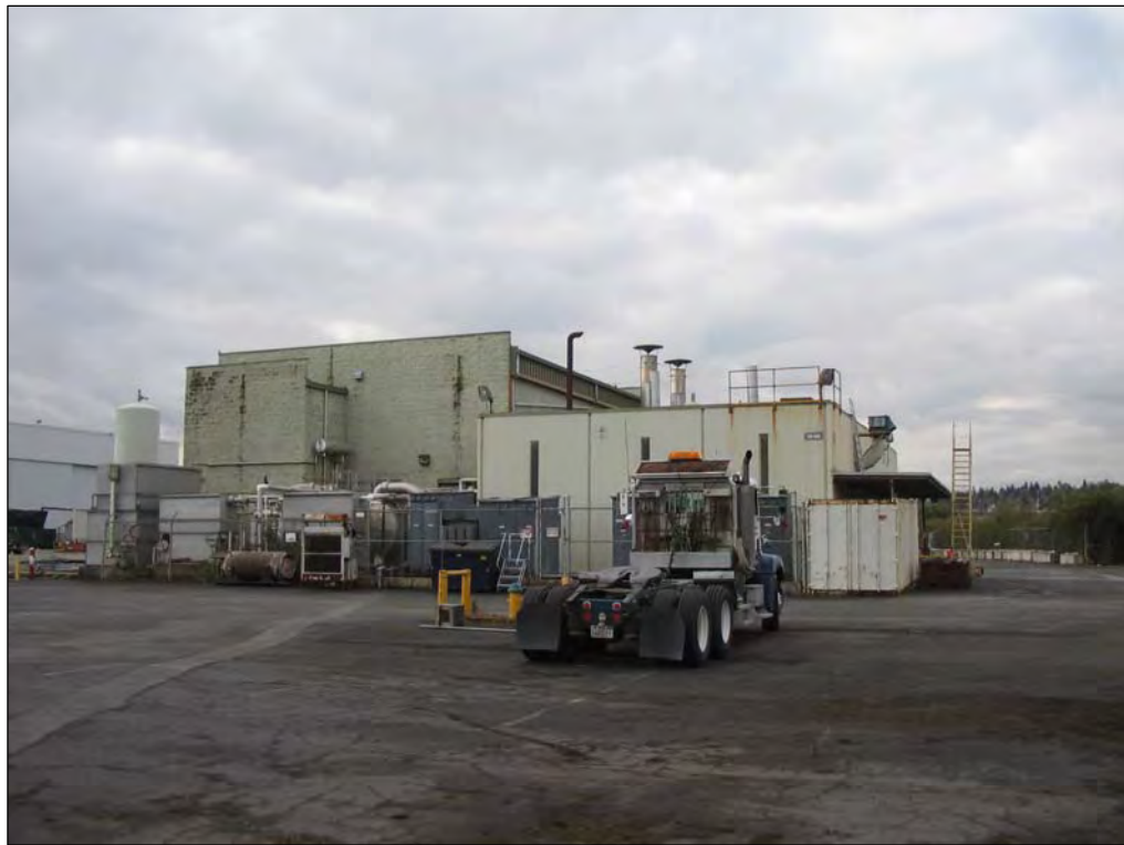
8. Looking south at Buildings 14-02 and 14-03.
