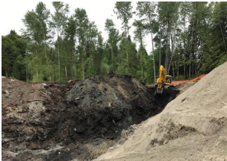
Excavation of landfill material from the wedge area
