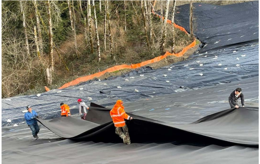
Installation of geocomposite drainage layer above 40-mil LLDPE geomembrane
