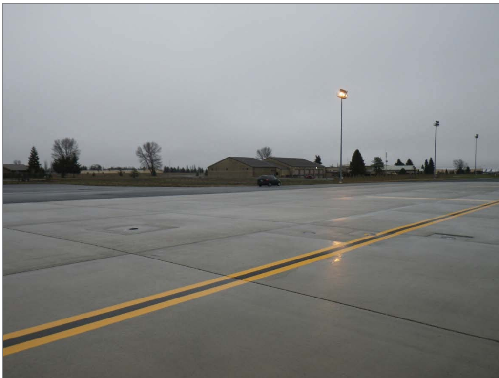
Photo 3. Site PS-2 (SS018) – Refueling Pit Area, looking north
