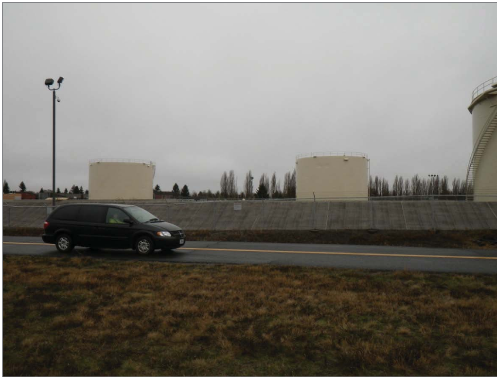
Photo 9. Site PS-1 (ST006) – Bulk Fuel Storage Area, looking west
