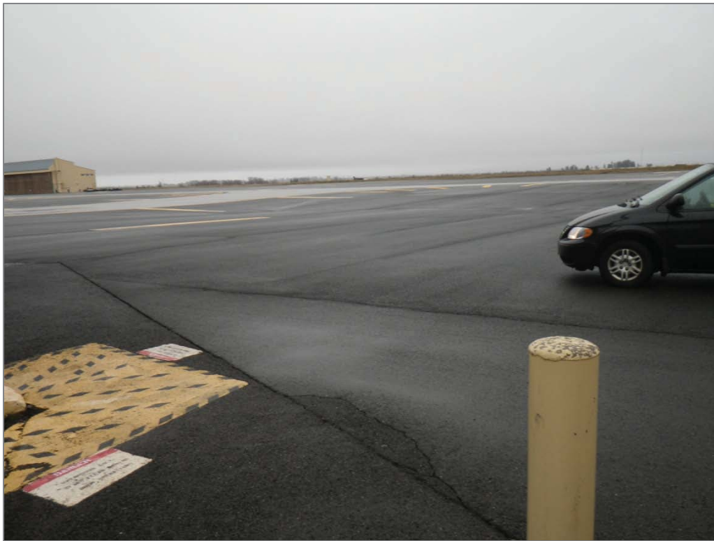
Photo 7. Site IS-3 (OT016) – Reciprocating Engine Test Cell, former Bldg 2150 area, looking south
