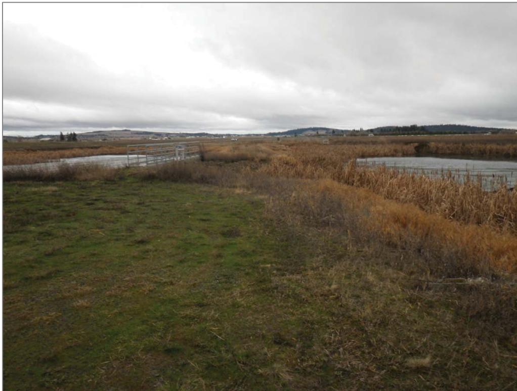
Photo 6. Site WW-1 (WP003) – Industrial Wastewater Lagoons (looking south between the holding lagoon on the left and the skimming lagoon on the right)
