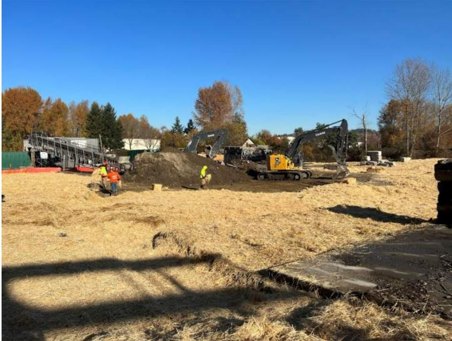
Photograph 27: Laying down straw for surface soil stabilization during final removal activities.
