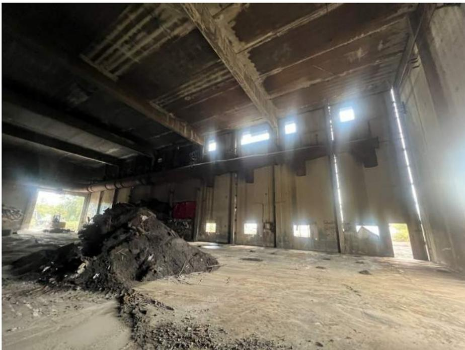
Photograph 14: Cleanup activities underway inside the building, baghouse hoppers removed and emptied. View to the south inside the building. 10/23/2023
