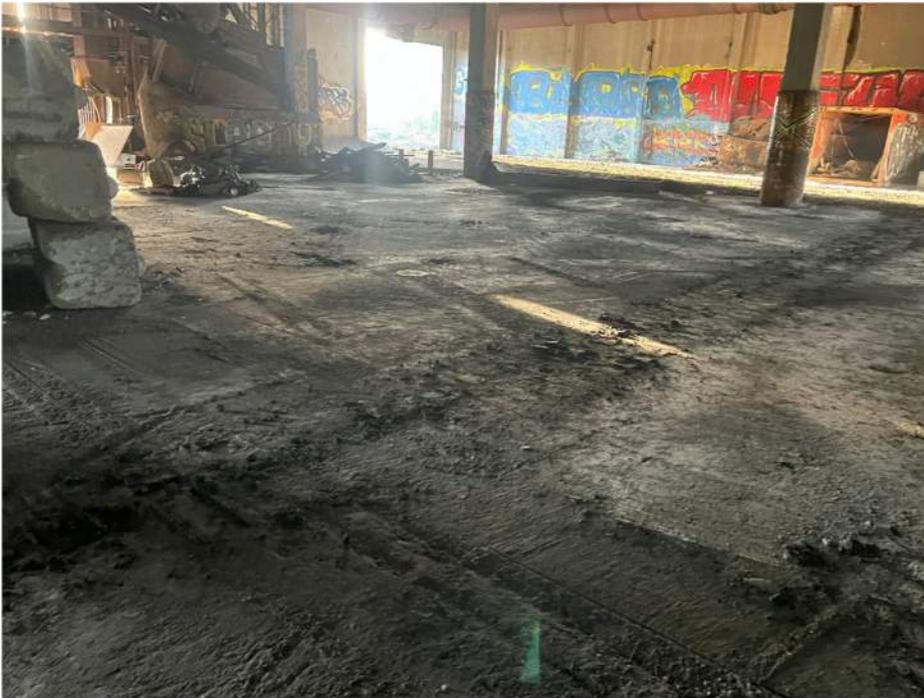
Photograph 12: Inside warehouse, dross removal and floor cleanup underway. View to the southeast inside the building. 9/29/2023
