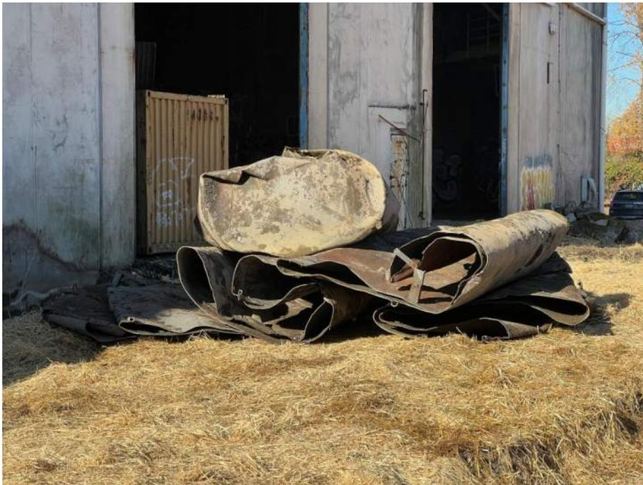
Photograph 26: Former open-top steel tanks, dross fines removed and tanks crushed for recycling. View to the northwest. 11/17/2023
