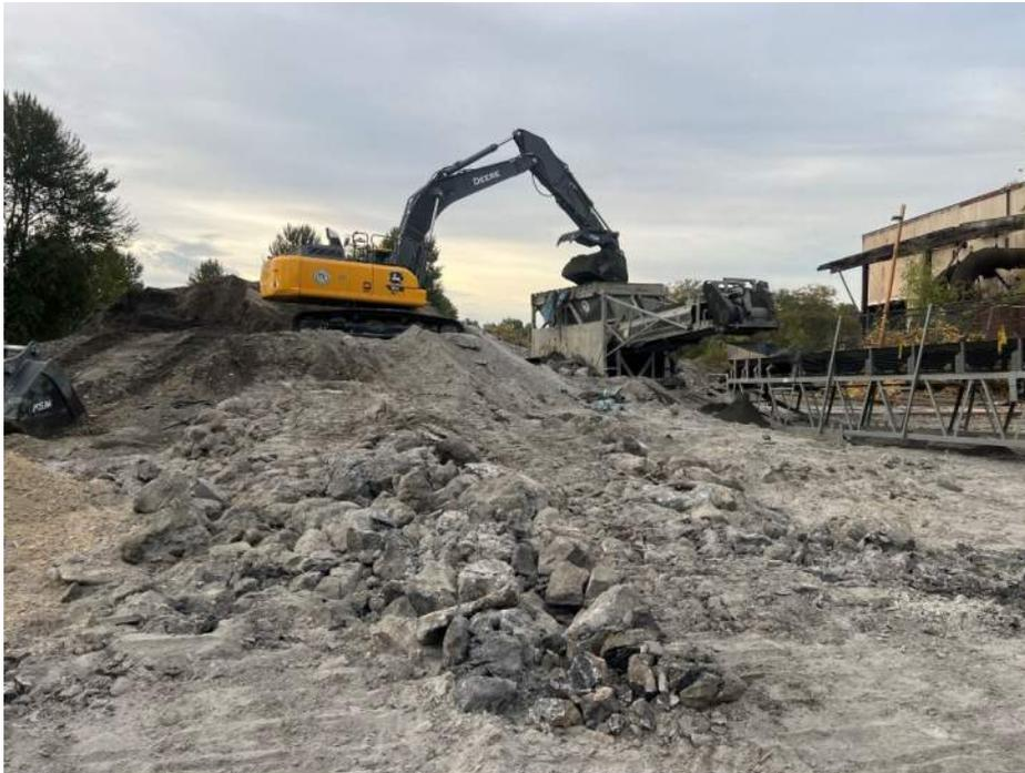
Photograph 8: Loading dross into hopper for conveyor system. Dross slag pile in the foreground. View to the south southwest. 9/11/2023.
