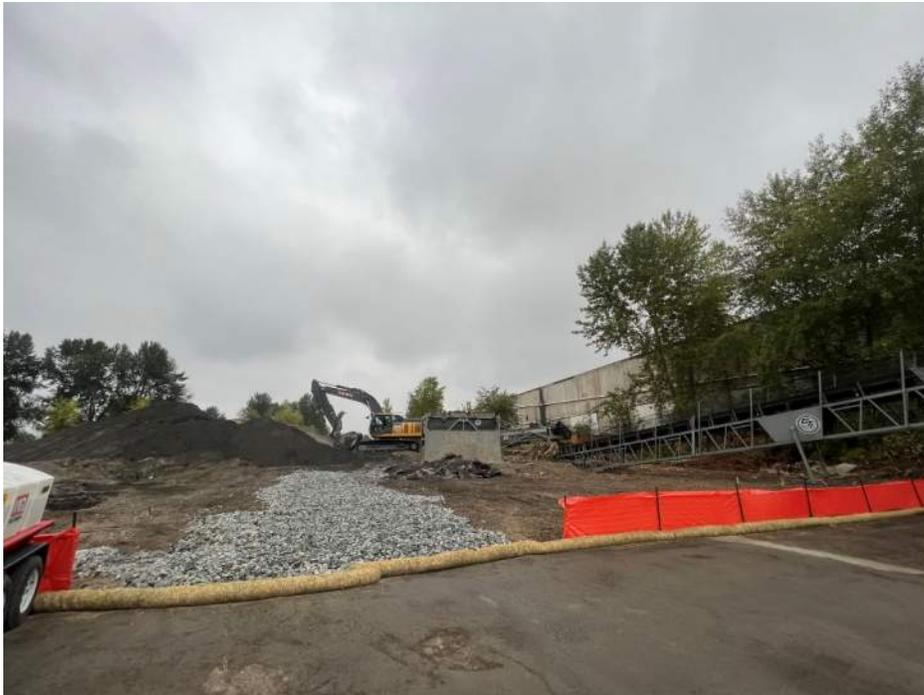
Photograph 6: Outdoor stockpile dross removal with TESC in place (stabilized construction exit, straw wattles on pavement, silt fence at soil perimeter). View to the south. 8/29/2023
