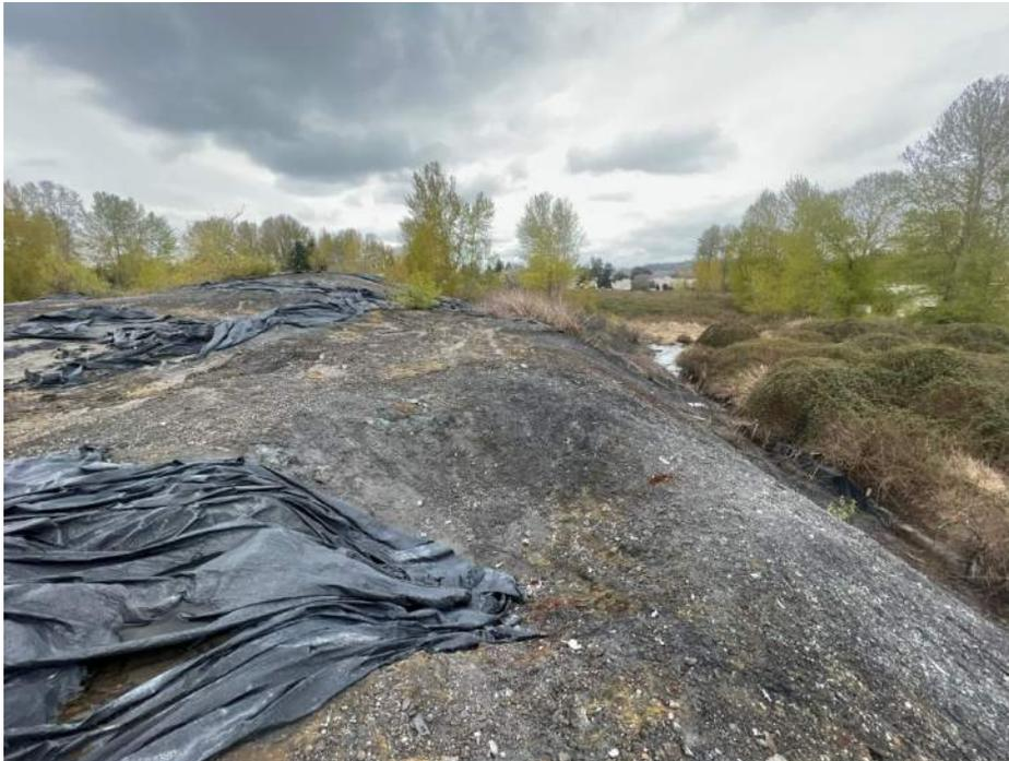
Photograph 2: Partial view of outdoor cross stockpile, view from on top of pile, geotextile cover deteriorated.
