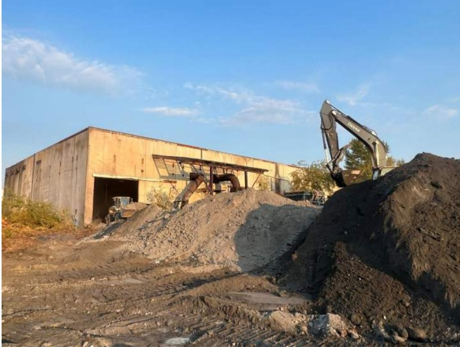
Photograph 11: Front-loader hauling indoor dross outside of warehouse to mix and load with outdoor dross, conveyor hopper in background. View to the west northwest. 9/22/2023
