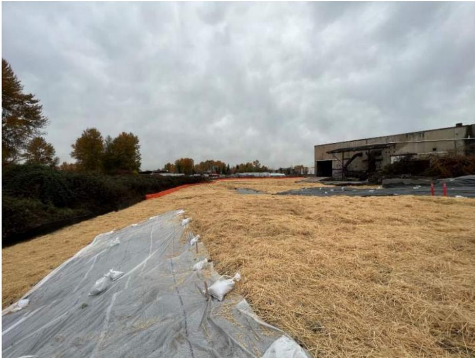
Photograph 22: Stabilizing site soil with straw and plastic sheeting (sloped areas) after drum removal. View to the south southwest. 11/9/2023
