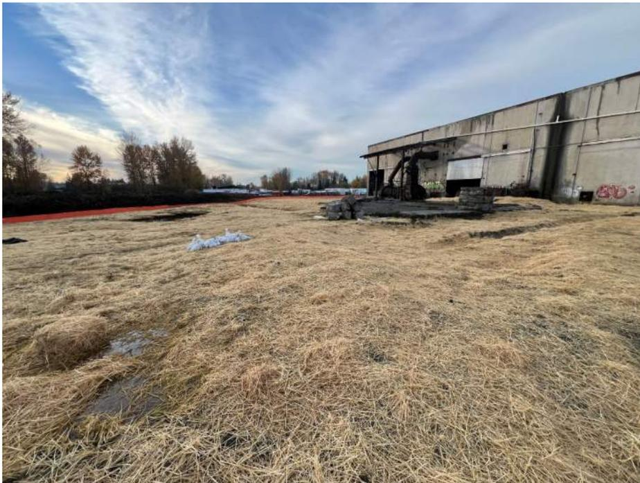
Photograph 28: Site conditions after bulk dross removal. Surface soil erosion controls in place (straw, plastic sheeting). View to the south. 11/21/2023
