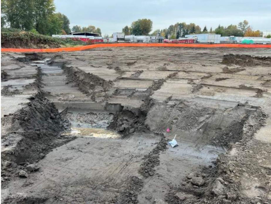
Photograph 21: Buried drum and drain pipe were removed (confirmation Sample CS-20 collected in this cell). View to the south. 11/1/2023
