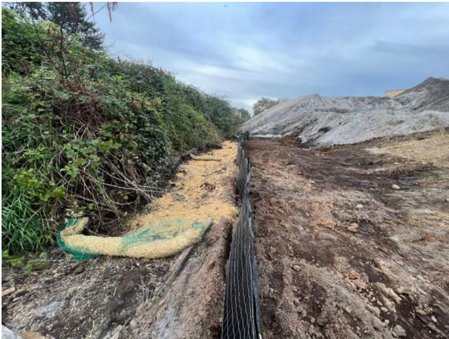
Photograph 10: Ditch conditions on the left, silt fence down the center and dross stockpile on the right. View to the southwest. 9/11/2023
