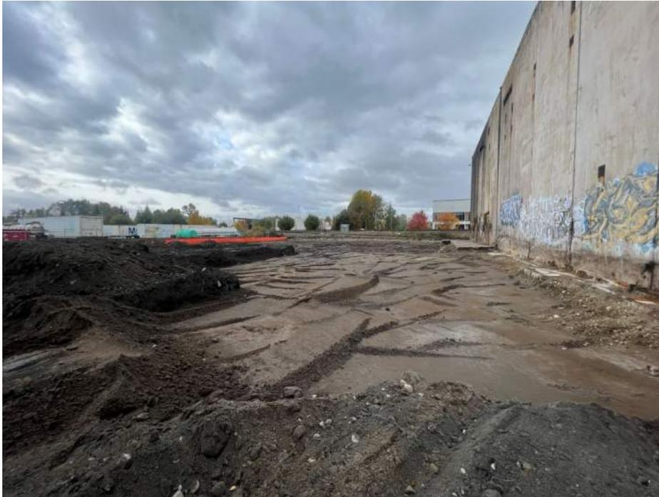
Photograph 15: Dross removal activities south of the building, ground surface exposed.
