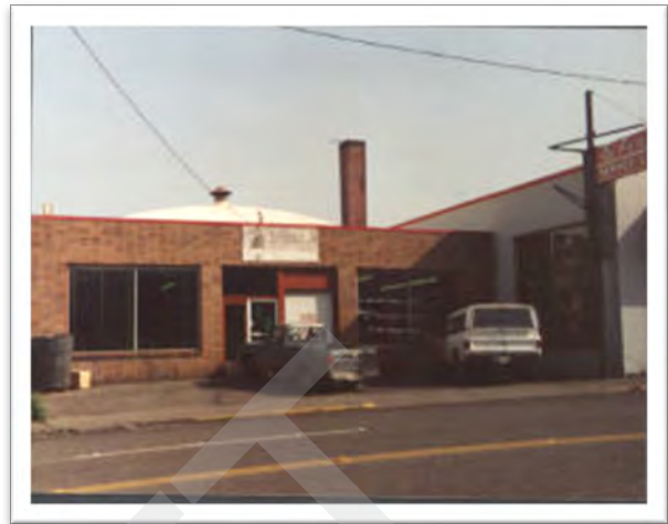
Photo 6-1. Circa 1970 photograph of the Williams Oil Filter Service Company building (1741 Jefferson Avenue).
