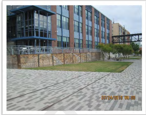
Photo 6-4. 2015 photograph of Science Building and final configuration of PLT looking northwest.
