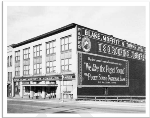
Photo 14-2. 1943 photo of TPS Building. (looking northeast).
