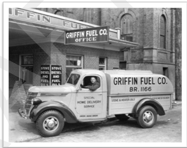
Photo 12-1: Circa 1940 Photograph of the Griffin Fuel Company office building in the foreground and the power distribution house in the background.
