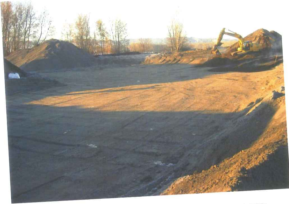
Spreading treated soil over Organoclay liner and compacting in 2' lifts
