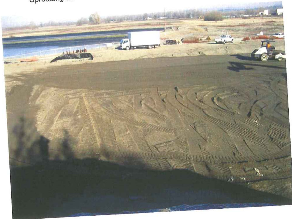
Spreading treated soil over Organoclay liner and compacting in 2' lifts
