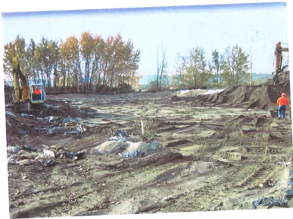
Removal of remaining treated soil to expose HDPE liner
