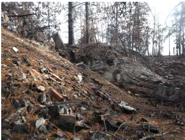
View of the Southeast End Area of the Large Building Materials Stockpile.
