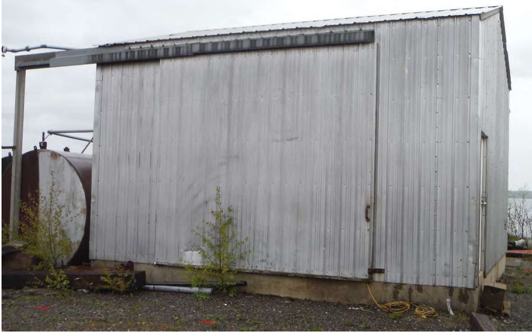
Photo 7 – Water Treatment Building Exterior
