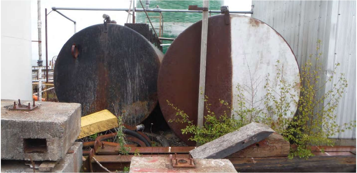
Photo 9 – Stormwater Tanks 7 and 8
