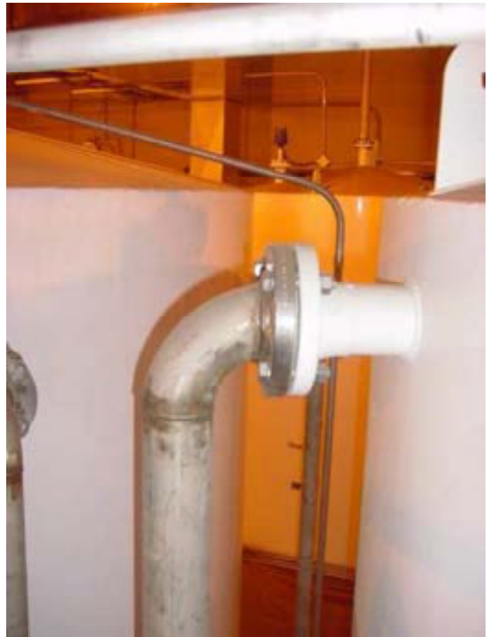
Figure 10. Tank 105 overflow pipe flange AOF-5.
