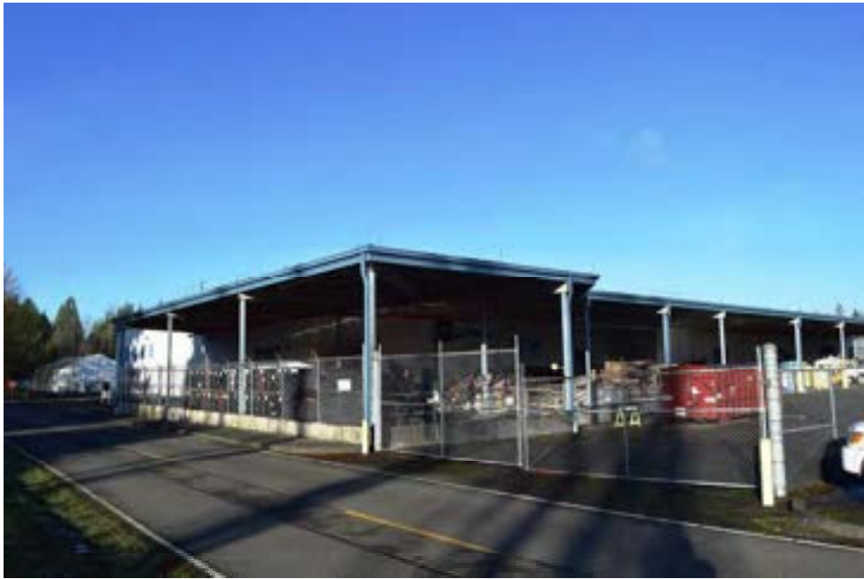
Photo 5: SE Corner, December 2017
