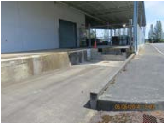
Pictures 5 & 6: the south loading dock spill containment area and associated sump.
