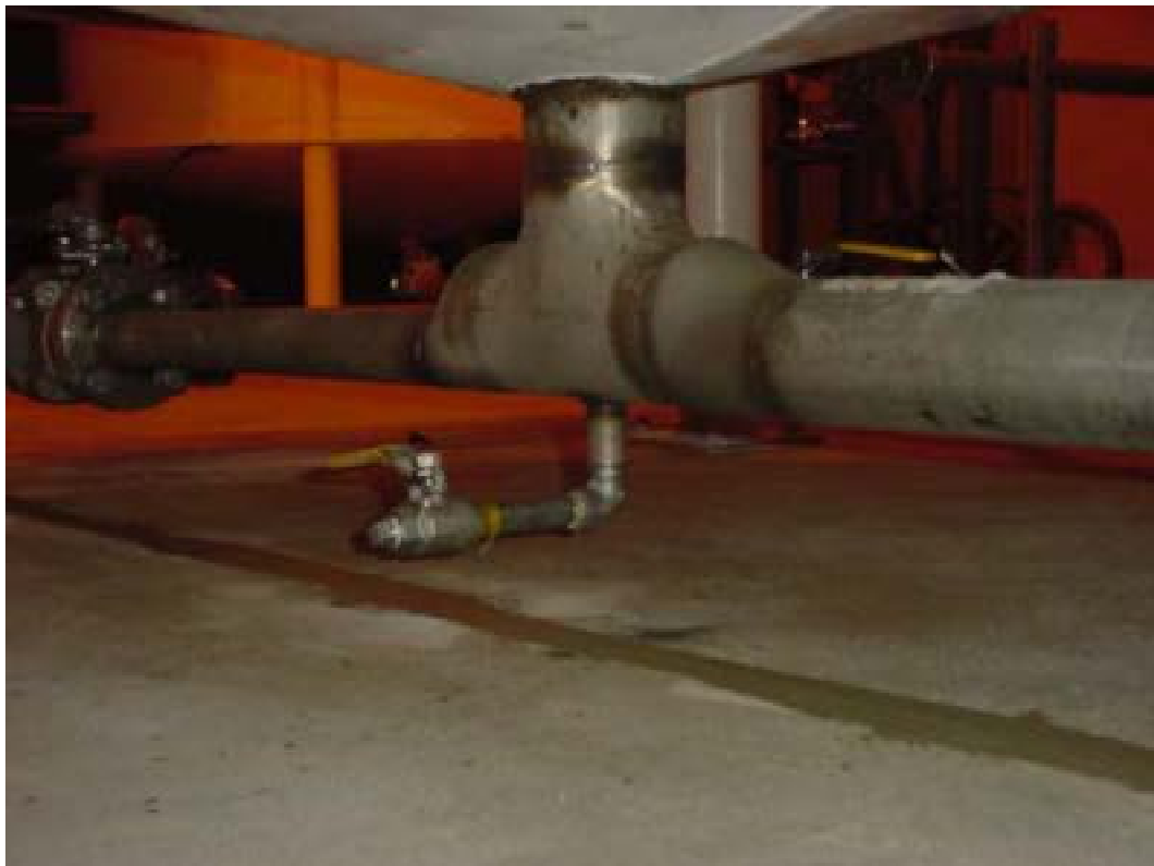
Figure 27. Tank 105 sample port valve AOV-7 and drain AOD-7. Test three threaded fittings and valve stem seal.
