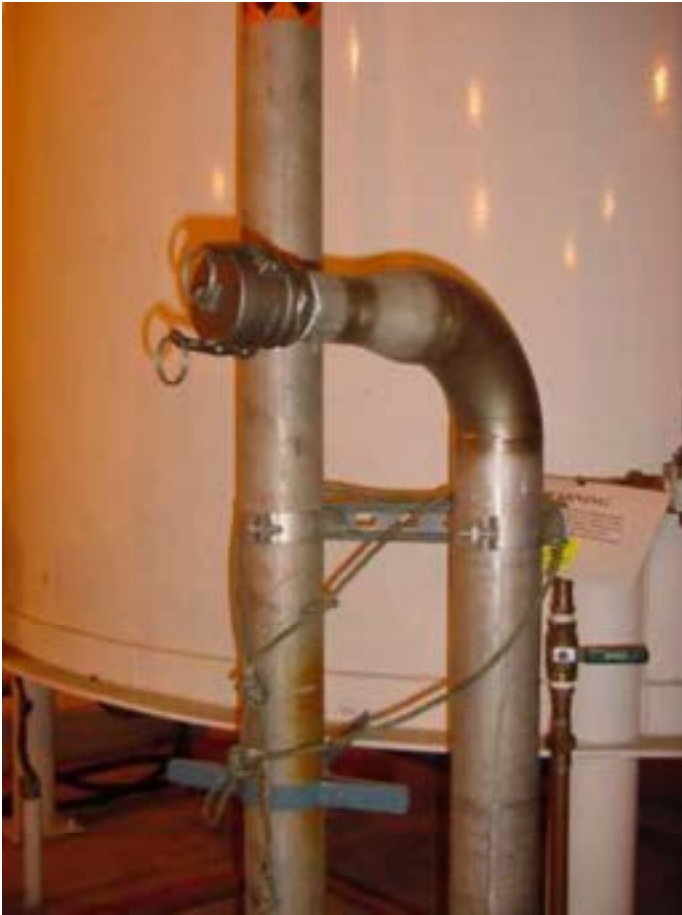
Figure 25. Tank 104 overflow end cap AOD-2.
