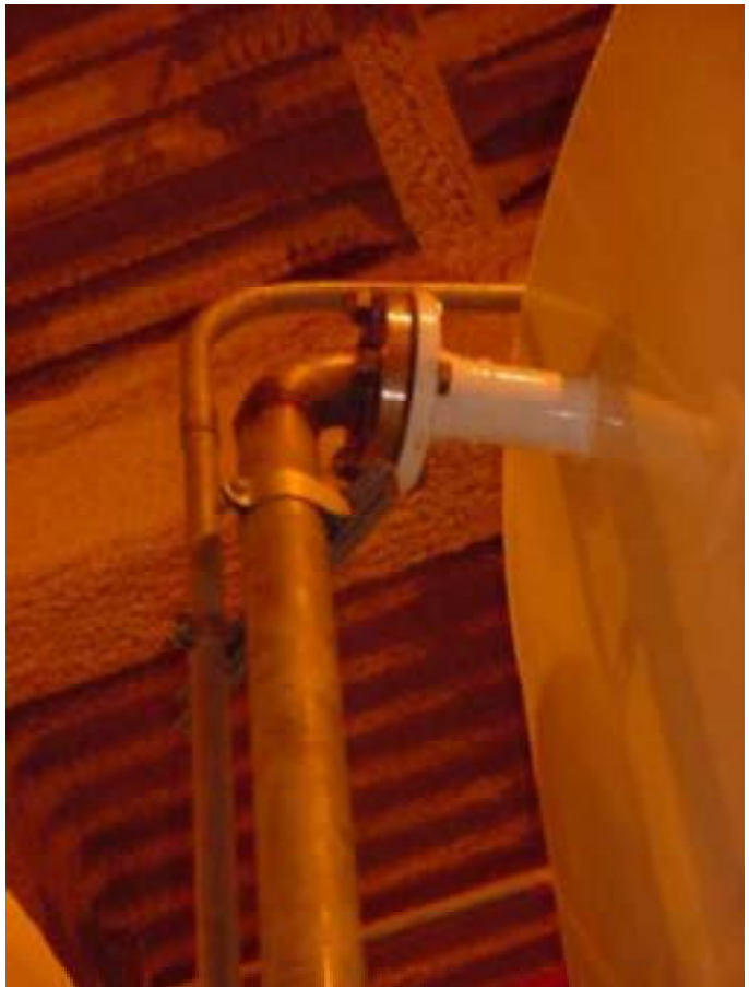
Figure 59. Tank 104 recirculation fill pipe flange ARF-8.
