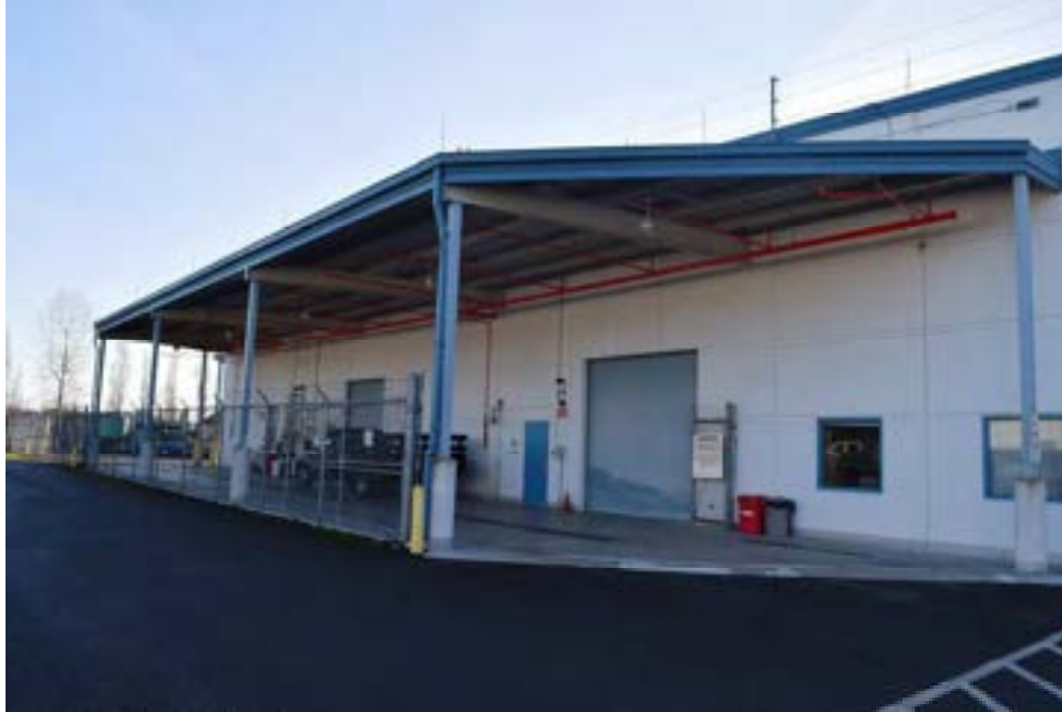
Photo 1: North Loading Area, December 2017
