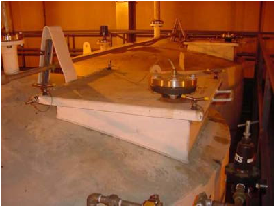
Figure 13. Tank 105 upper access hatch cover AIF-4. Test underside of entire hatch perimeter.
