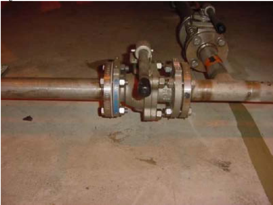
Figure 43. Recirculation drain flex hose flange (to be deleted in upgrade). Test perimeter of flange.
