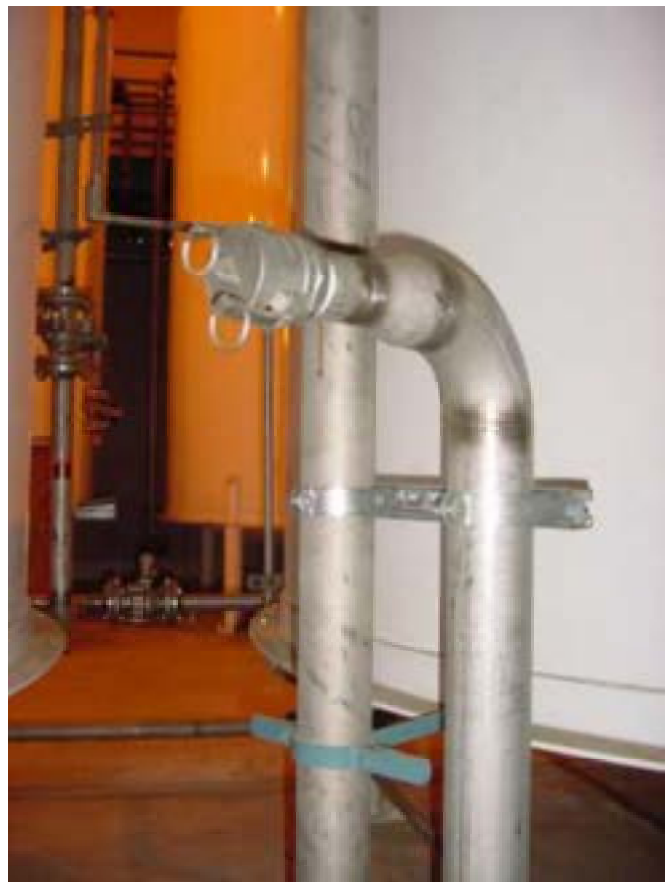
Figure 26. Tank 105 overflow end cap AOD-5.
