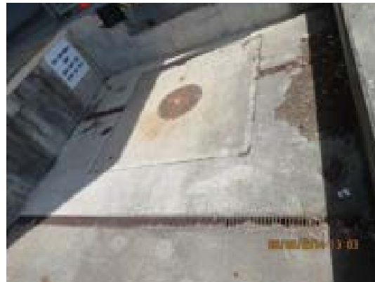
Pictures 5 & 6: the south loading dock spill containment area and associated sump.
