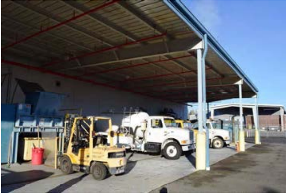
Photo 7: East Storage Area, December 2017
