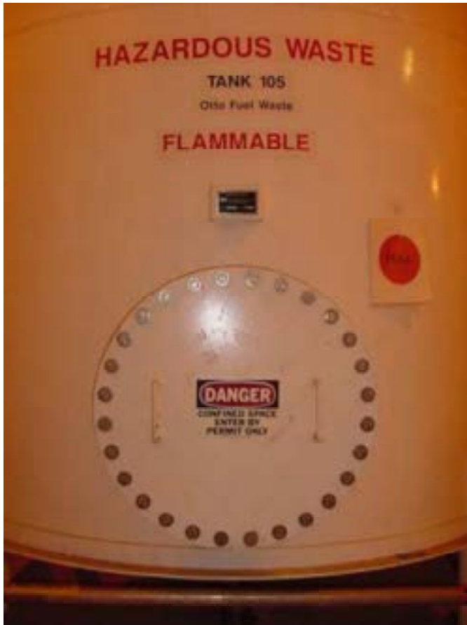
Figure 35. Tank 105 bottom access cover AOF-6.
