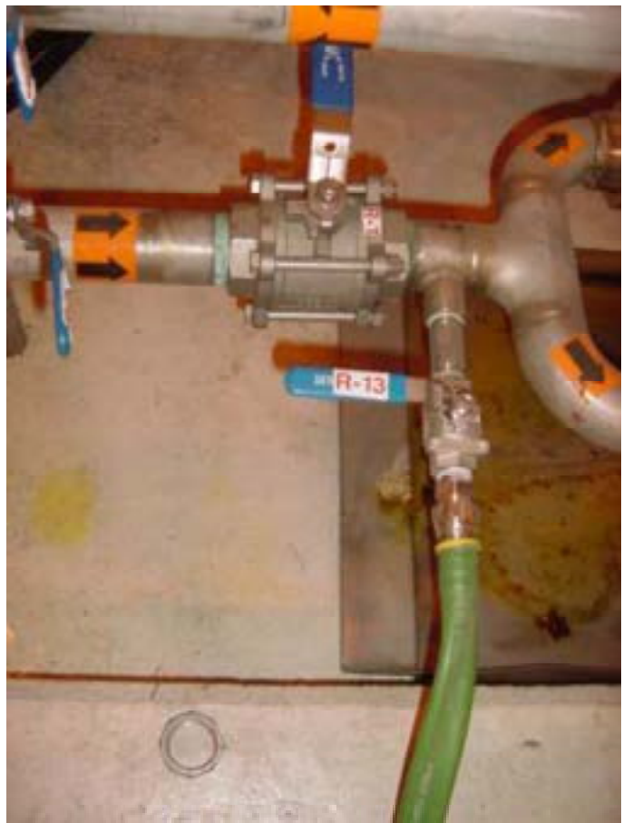
Figure 48. Recirculation drain valves ARV-1, sample port valve ARV-2 and drain sample port ARD-1.
