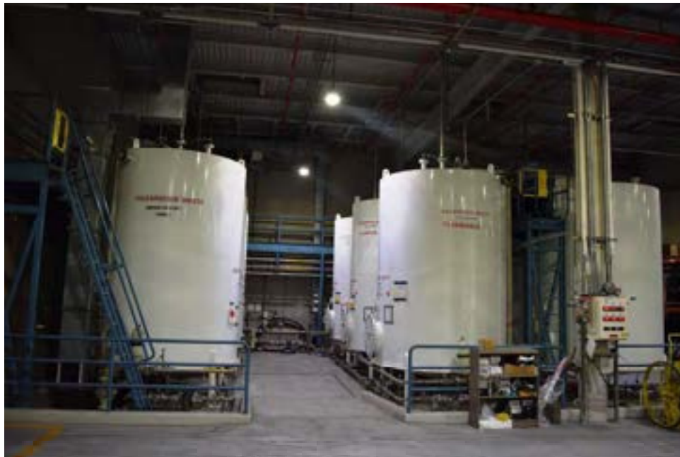
Photo 14: Tank Storage Area (Rm 124), December 2017
