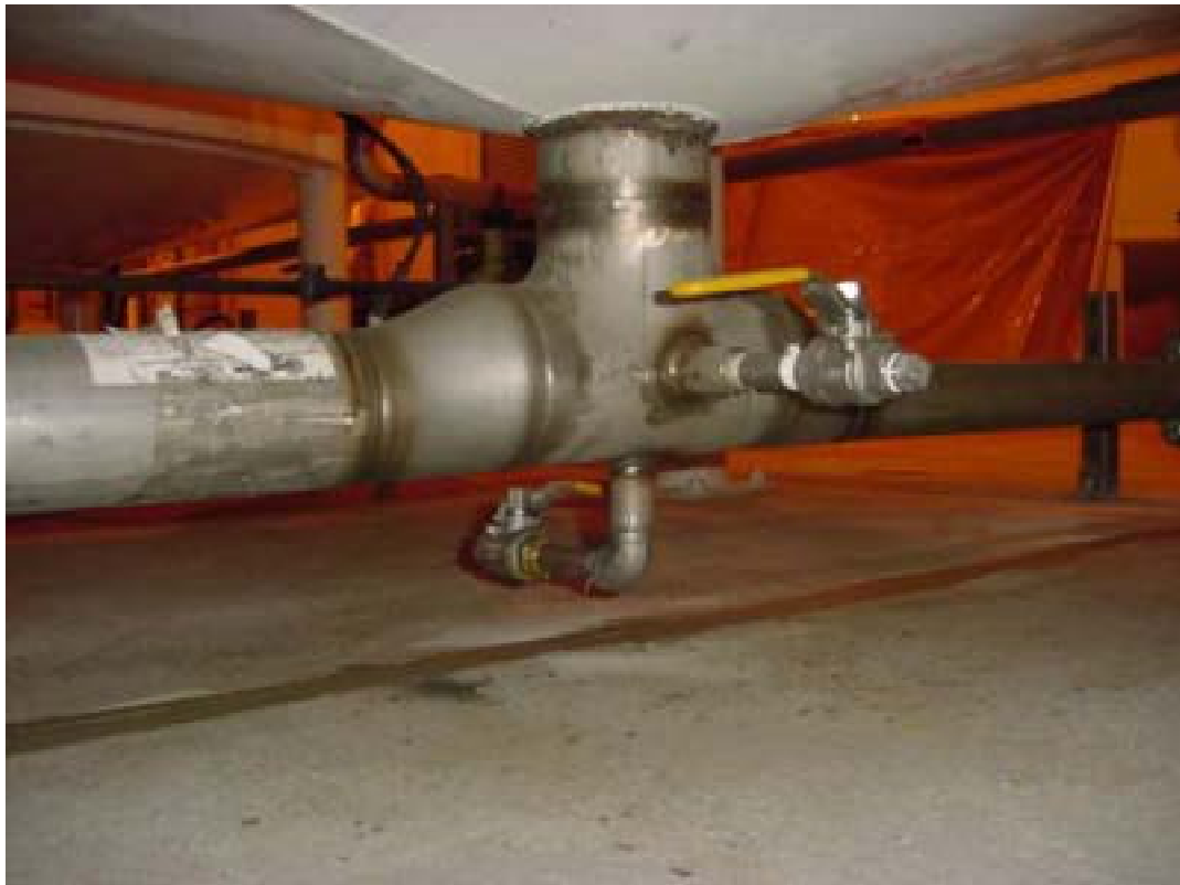
Figure 27. Tank 105 sample port valve AOV-7 and drain AOD-7. Test three threaded fittings and valve stem seal.
