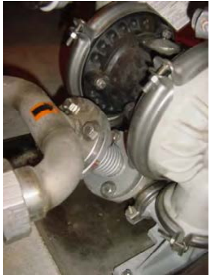
Figure 52. Recirculation drainpipe flex fitting ARF-3.
