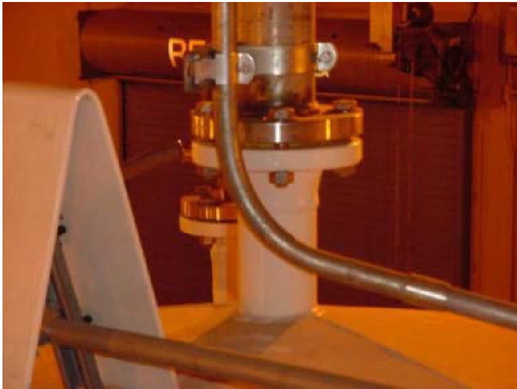
Figure 5. Tank 104 vent flange AOF-1. Test perimeter of vent flange.
