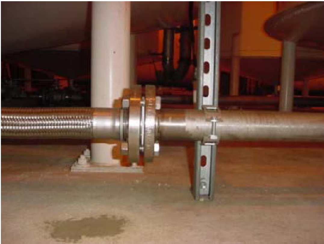
Figure 43. Recirculation drain flex hose flange (to be deleted in upgrade). Test perimeter of flange.
