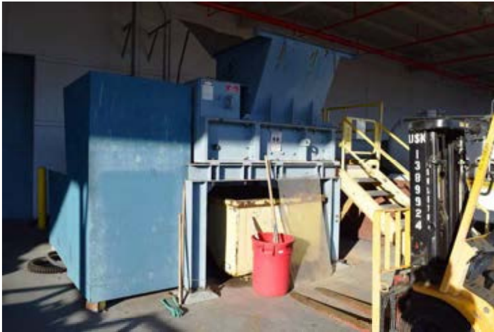
Photo 8: Drum Shredder, December 2017
