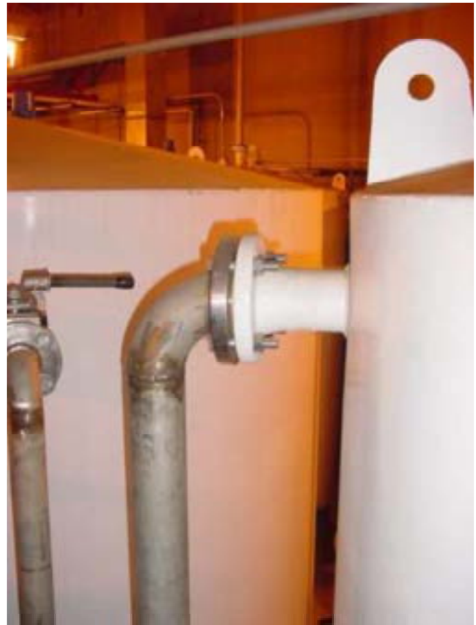
Figure 16. Tank 106 overflow pipe flange COF-5.
