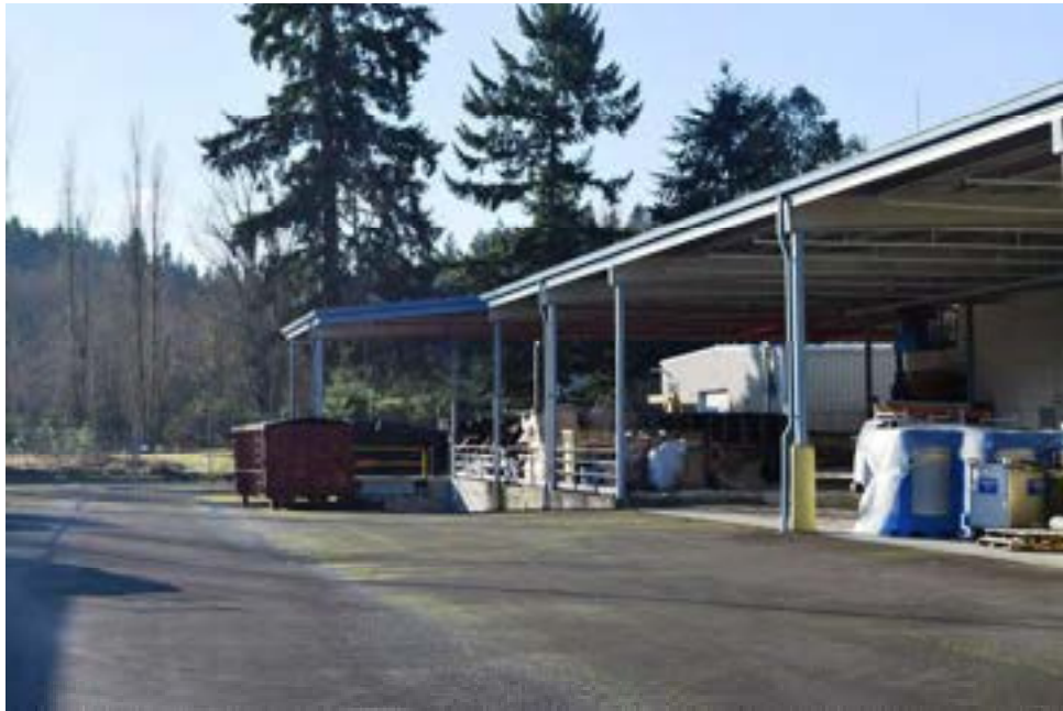
Photo 6: SE Storage Area, December 2017
