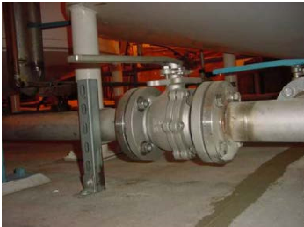
Figure 30. Main drain pipe valve AOD-5. Test perimeter of flanges at either end of valve, valve center flange, and valve stem seal.
