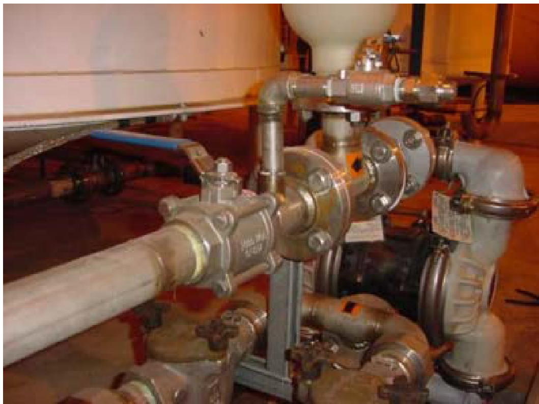
Figure 55. Recirculation fill valve ARV-4, fill sample port valve ARV-3, and sample port ARD-2. Test perimeter of both ARV-4 flanges and threaded fittings, four ARV-3 threaded fittings, both valve stem seals and sample port.
