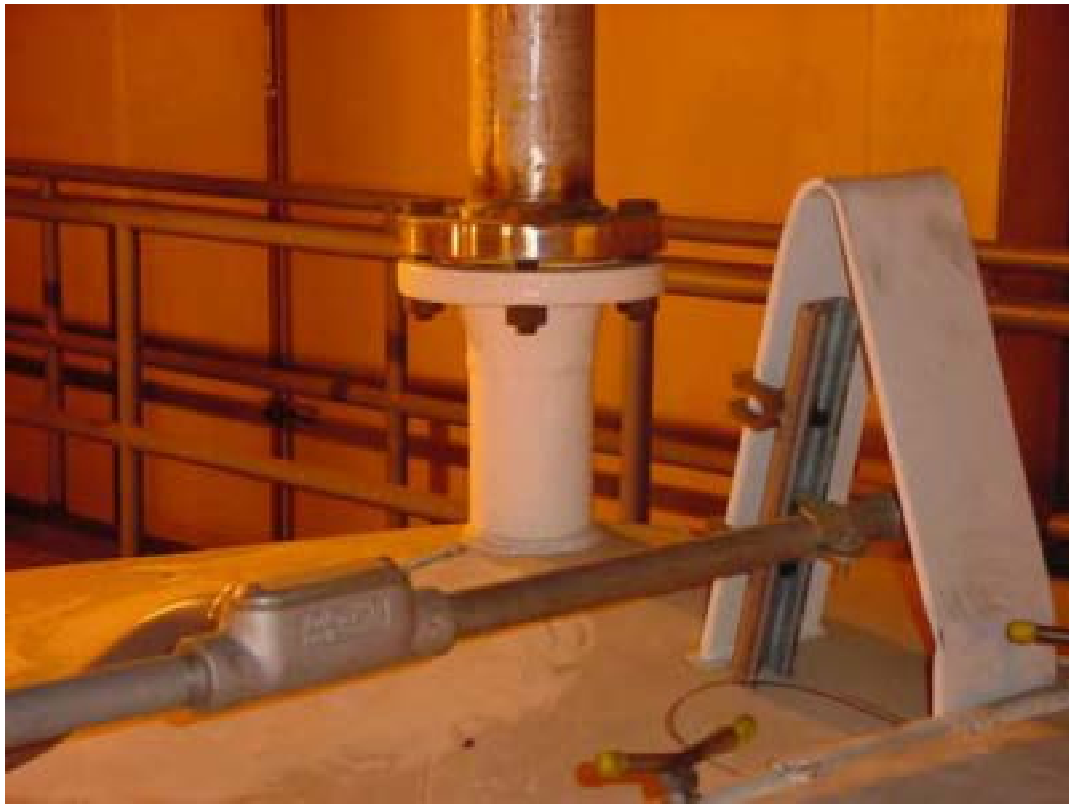
Figure 17. Tank 106 vent flange COF-4. Test perimeter of vent flange.
