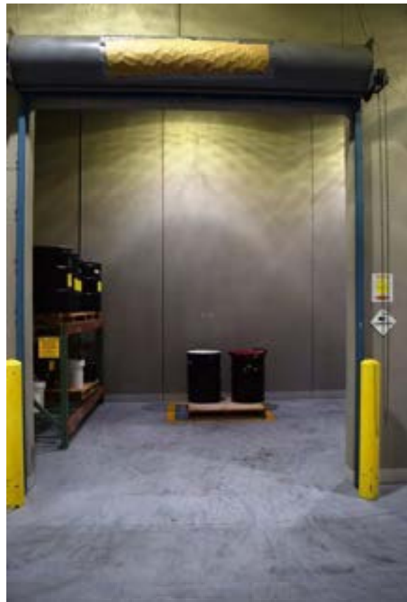
Photo 24: Alkaline Room (Rm 138), December 2017
