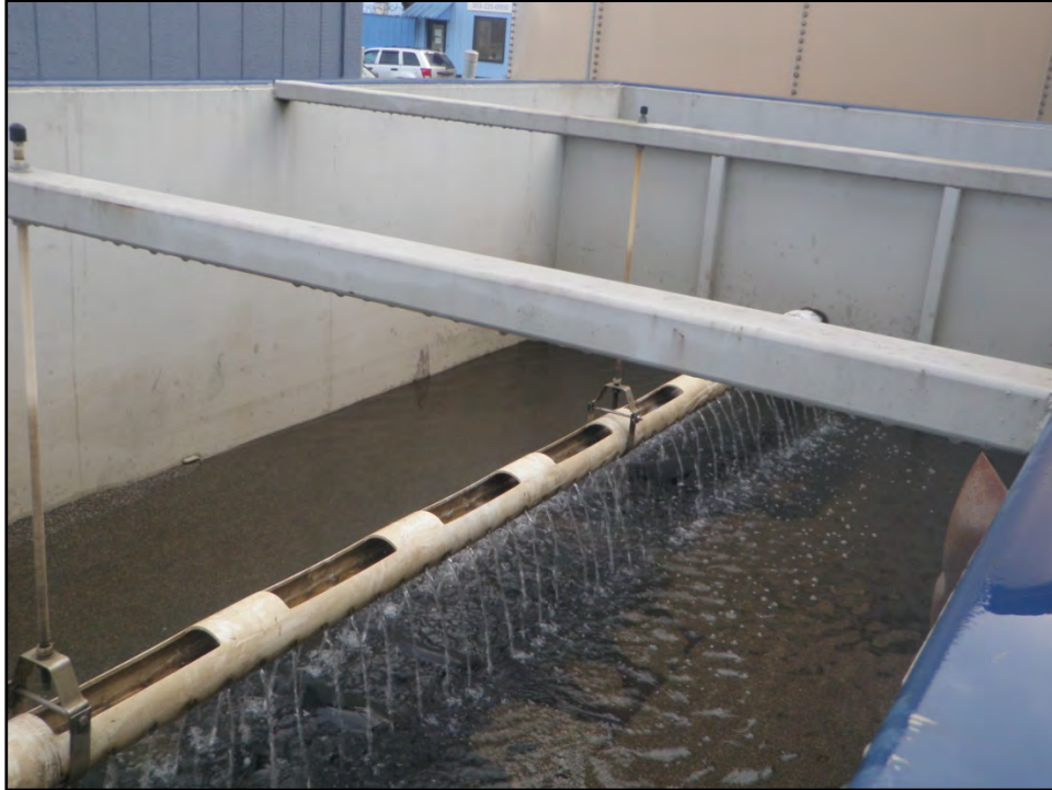
Figure 6. Best operating water level in filtration chamber for optimal pollutant removal conditions
