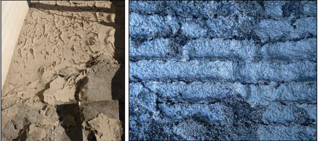
Figure 5. Accumulation of solids on the media bed surface
