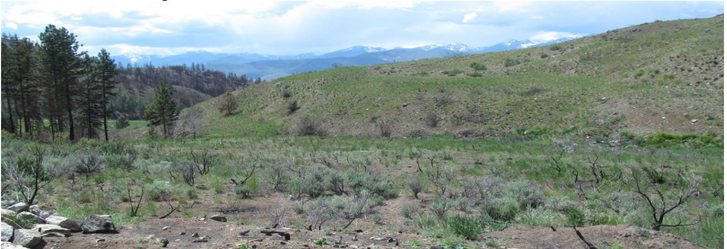
Minnie Mine – General Cap Condition from the North
