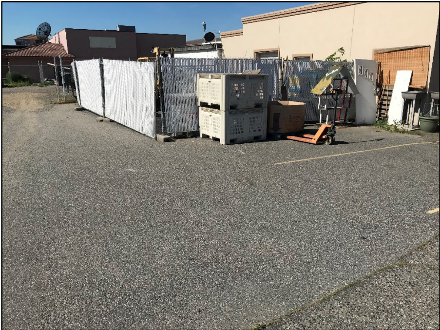
Photo 4: Fenced area on east side of structure (view to southwest)
