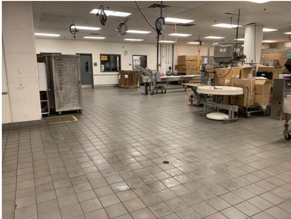
Photo 10: Concrete core location of borehole B4
