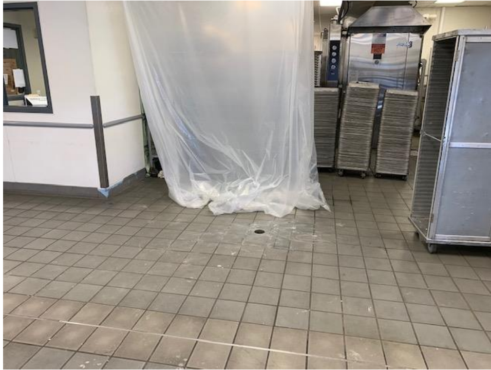
Photo 3: Location of borehole B1
