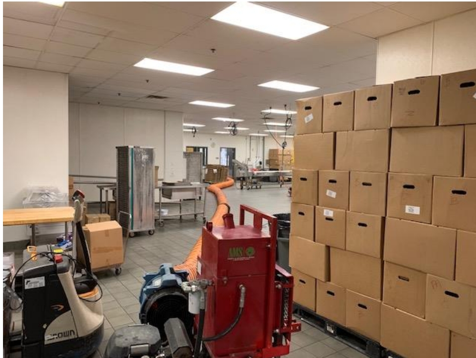
Photo 8: Venting system leading exhaust to exterior
