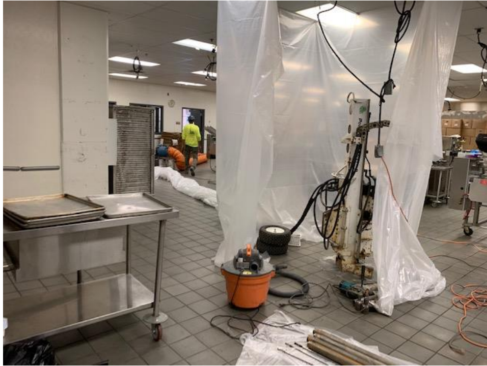
Photo 7: Location of borehole B2
