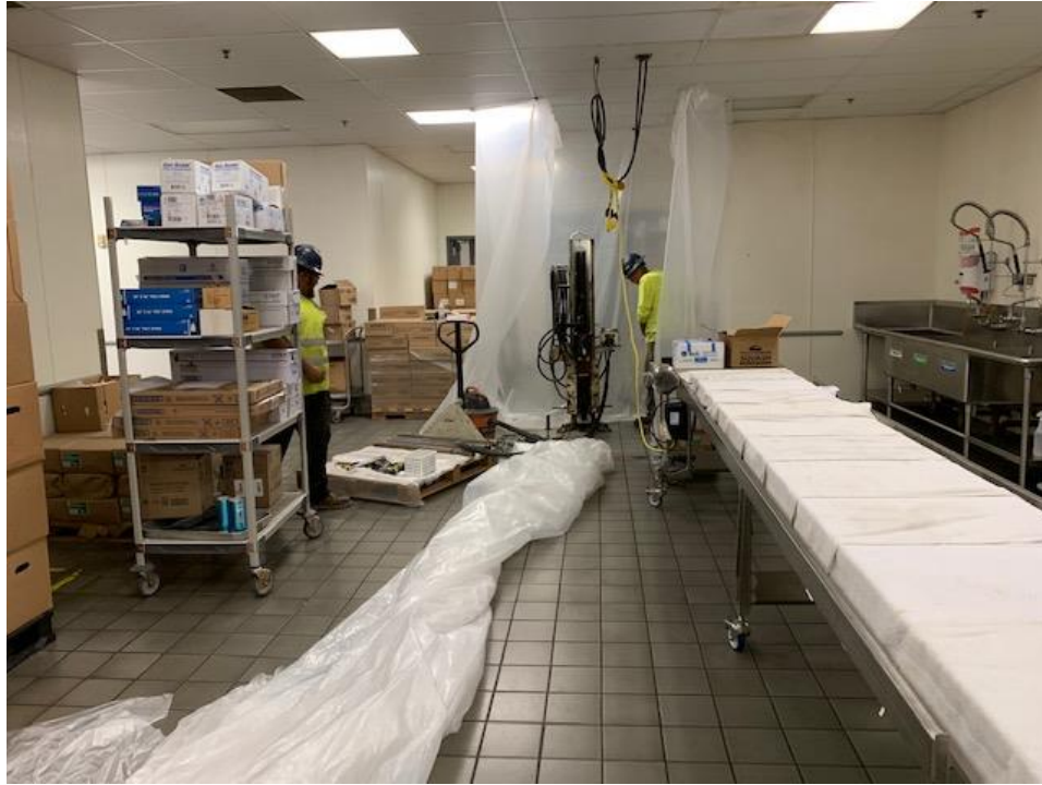
Photo 9: Location of borehole B4 and protective plastic
