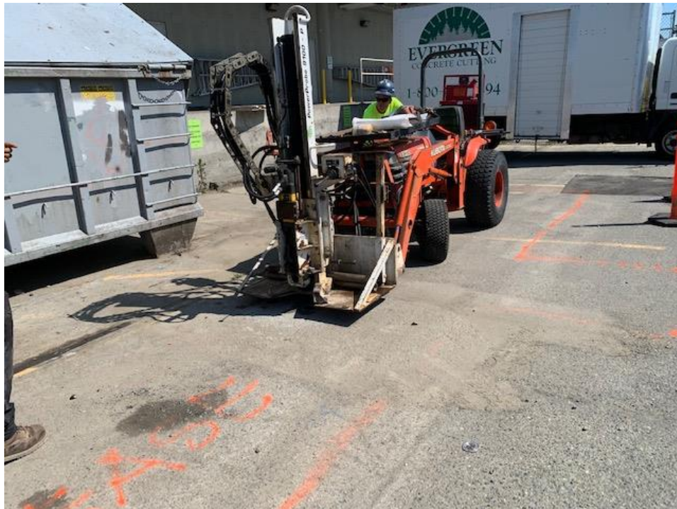
Photo 2: Dolly mounted drill rig
