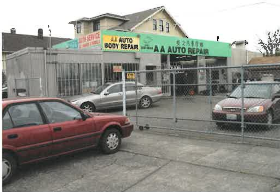
1. Looking southwest at the subject site and building
