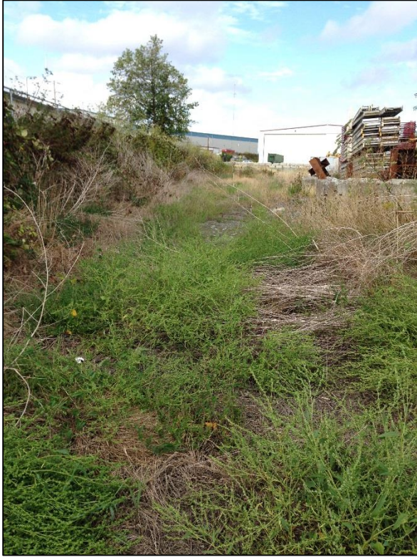
Photograph A-7 – Photo point 4 drainage swale
