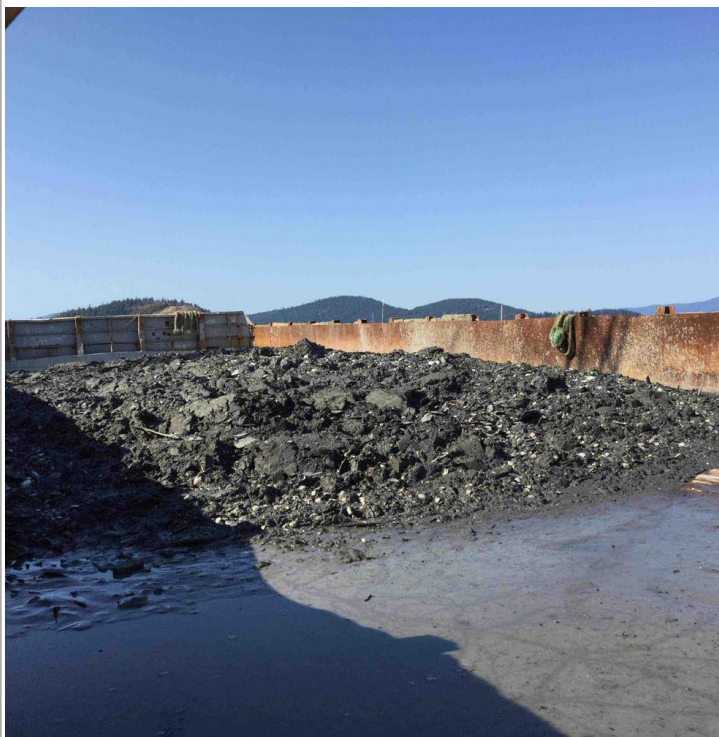
Dredge materials to date (7-27 thru 7-29).
