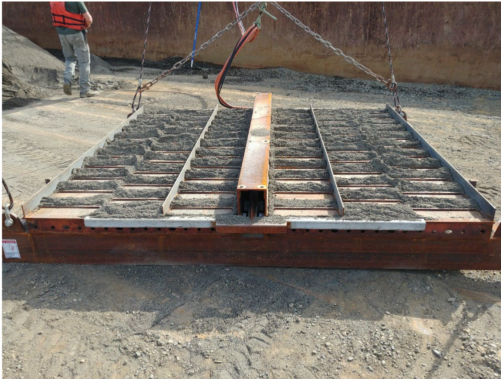
Photo #11: Steel table used to uniformly deposit the 2-inch thin layer cap, located on the barge with a small amount of material remaining after deposition
