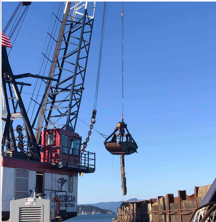
Pile removed from north dredge prism.
