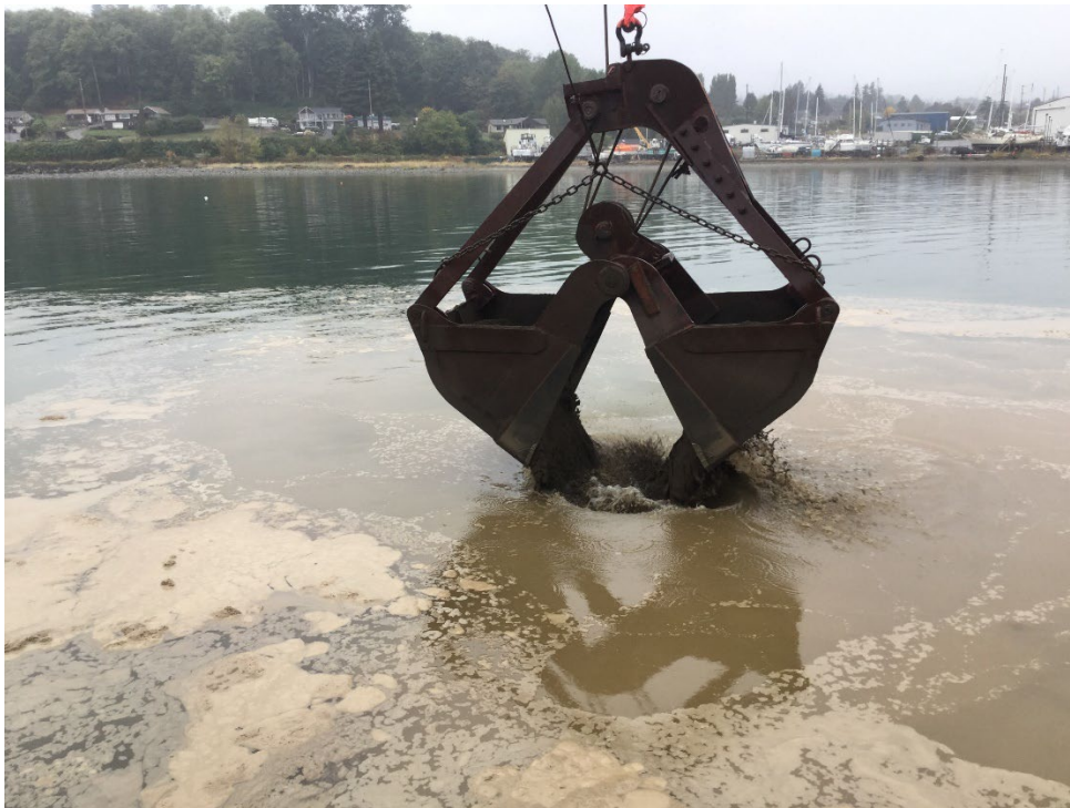
Photo #8: Clamshell bucket backfilling material close to the surface of the water.
