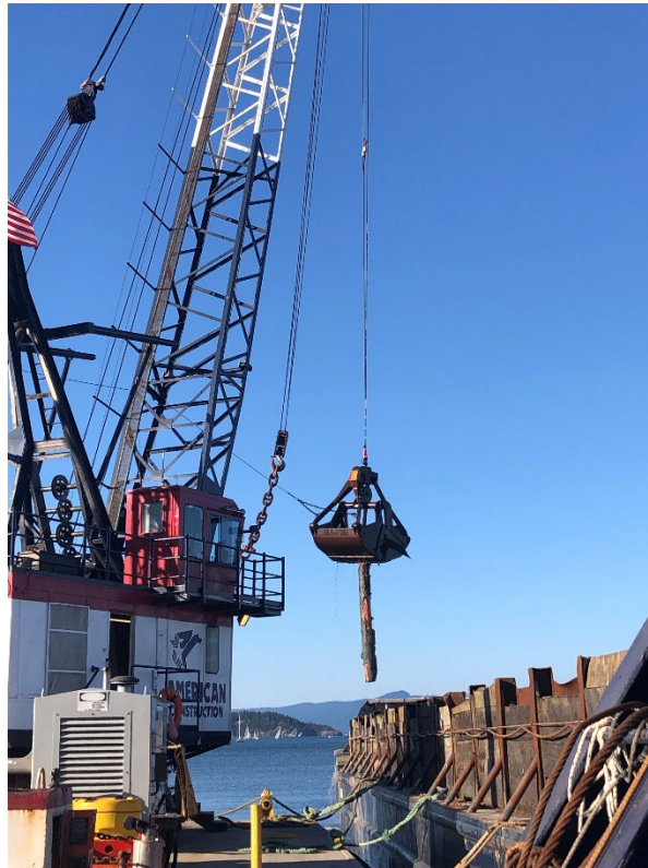
Photo #7: Clamshell bucket removing anomalous debris (derelict pile) encountered during dredging.
