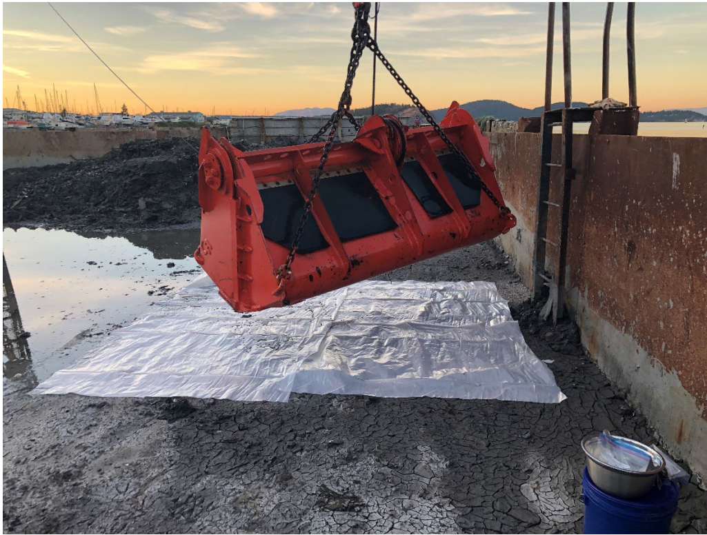
Photo #3: Environmental bucket utilized during dredging with plastic sheeting laid down for sampling purposes
