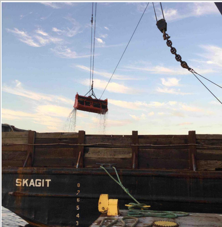
Environmental bucket over barge
