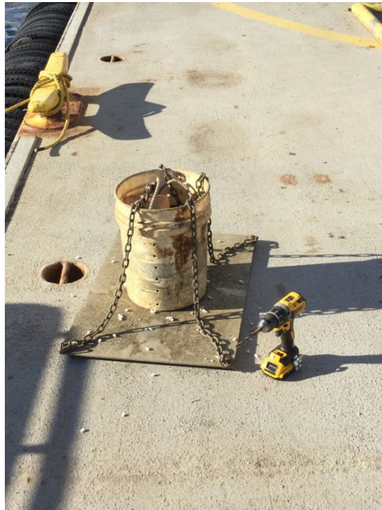
Photo #9: Rain bucket utilized to approximately measure the thickness of backfilled material as it was placed.
