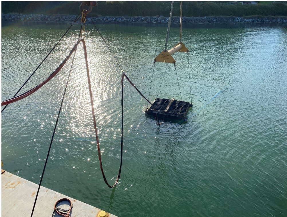
Photo #15: Backfill underway utilizing the 2-inch thin layer cap steel table.
