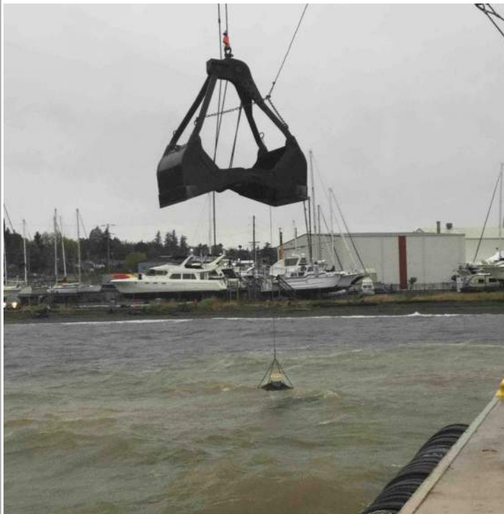
Crane pulling rain bucket.
