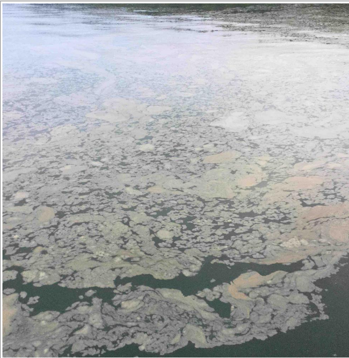
Film of fines from 8" TLC material and entrained air resulting from placement with 4 CY bucket.
