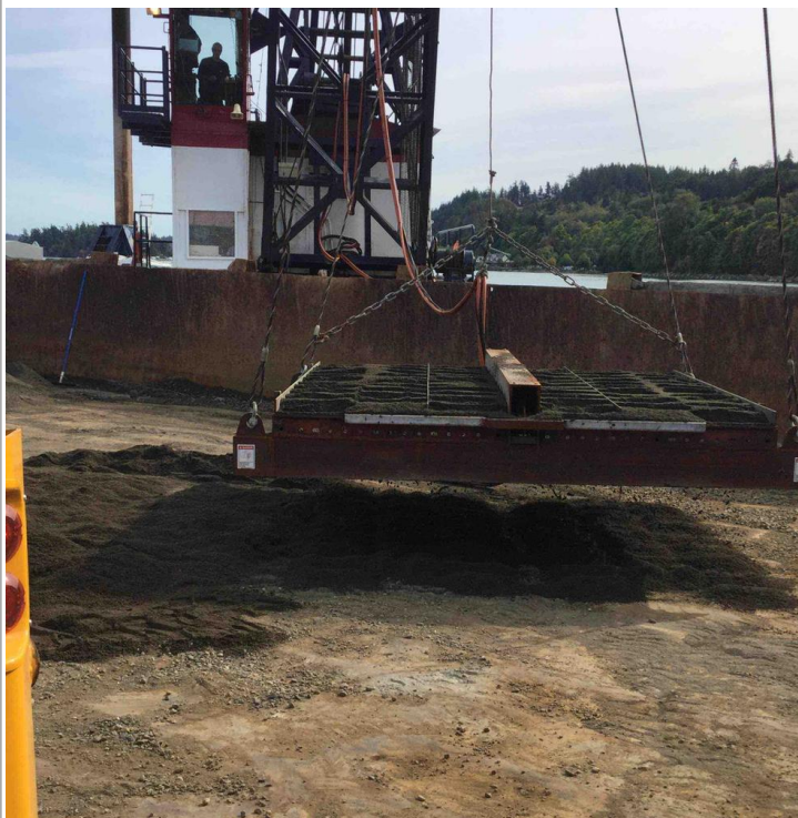
Dry run on deck with overlap between sets. This run assumed the table distribution would be a 9'x9' square
