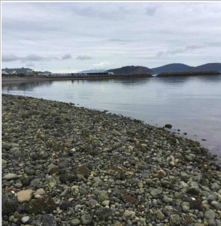
Beach prior to the start of work, adjacent to yesterday's areas of activity.
