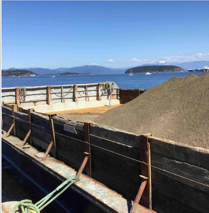
Full materials barge, start of day. (1 of 3)
