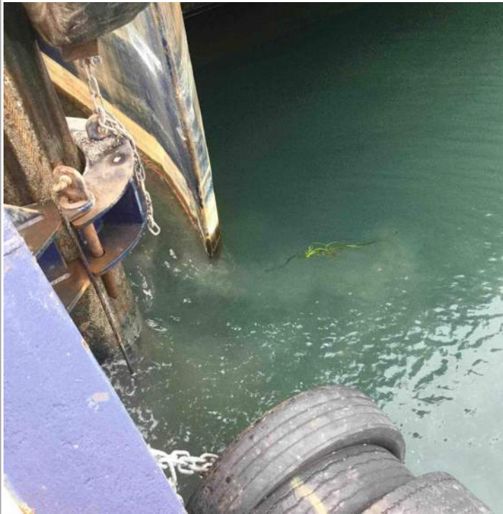
Damaged eelgrass from spud placement.
