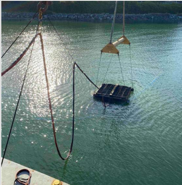
View from crane of table placing the 2-inch TLC.
