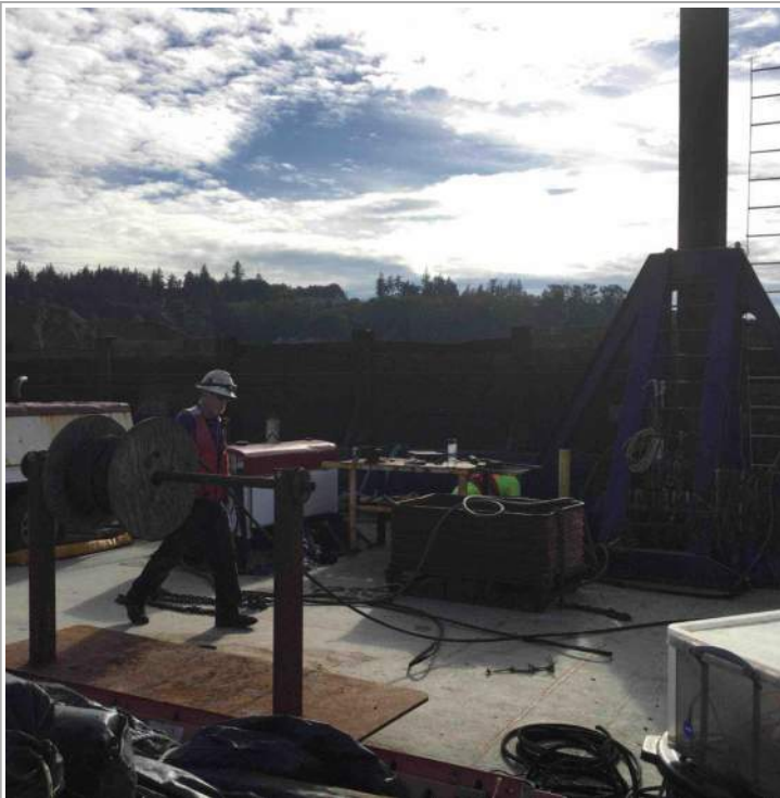
Crew replacing spud cable.
