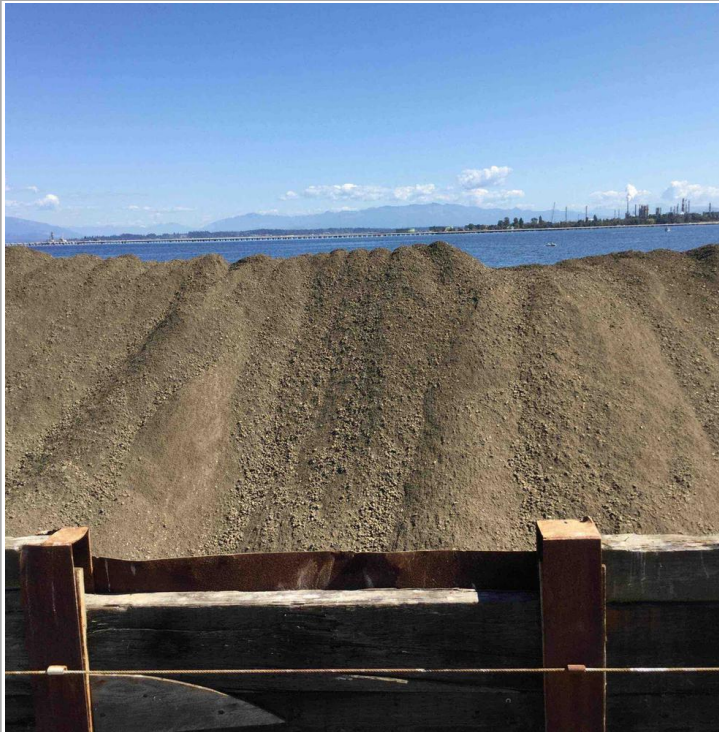
Full materials barge, start of day. (2 of 3)
