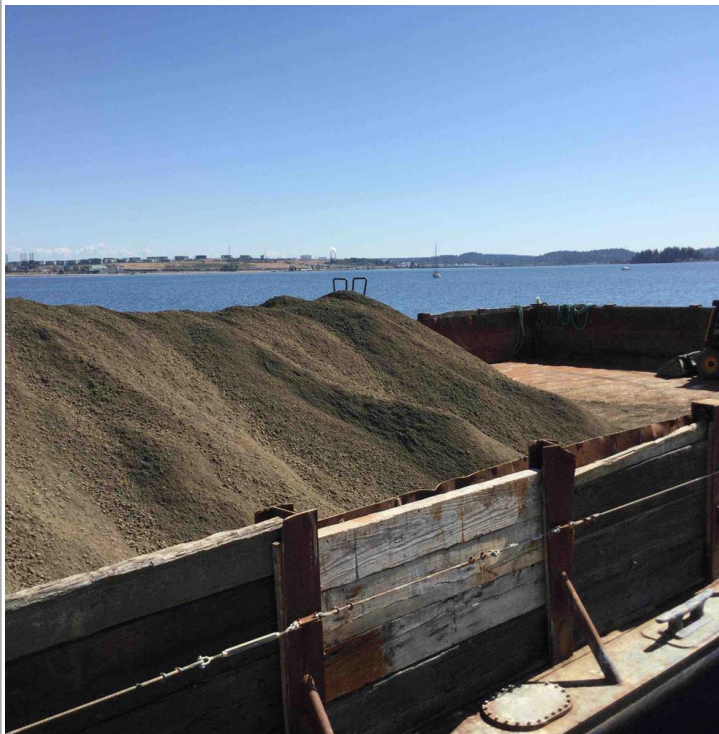
Full materials barge, start of day. (3 of 3)
