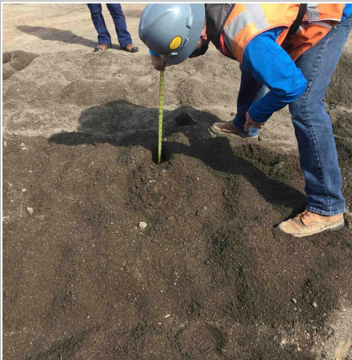
John measuring depth of dry run on deck.
