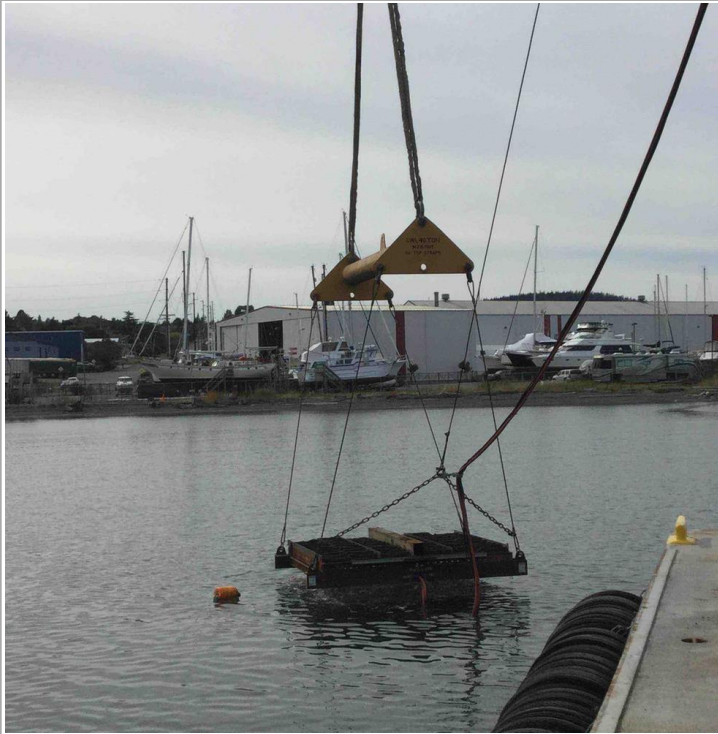
"Wet run" testing placement with an added bucket and survey.
