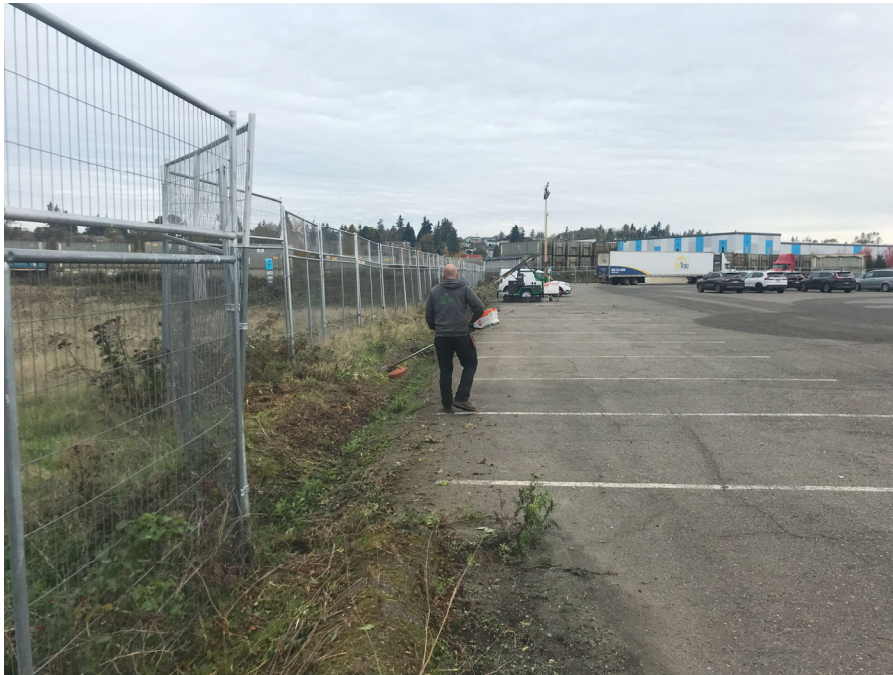
Photograph 3 – Looking west at southeastern portion of the asphalt cap. Photograph shows landscaping crew removing vegetation from the south drainage ditch. Vegetation was observed to be growing through minor cracks and adjoining soil cap area.
