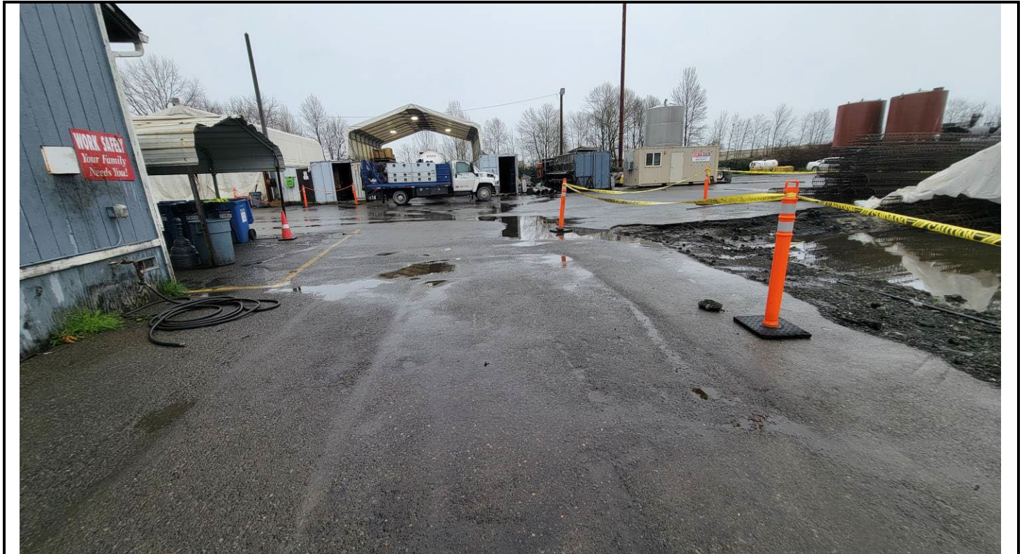
South portion of truck route, looking east, near adjacent to former UST removal area (under lunchroom building).
