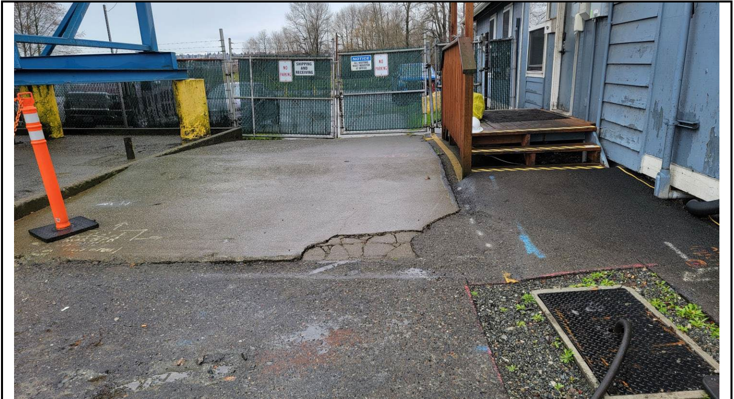
South exit gate concrete pad.
