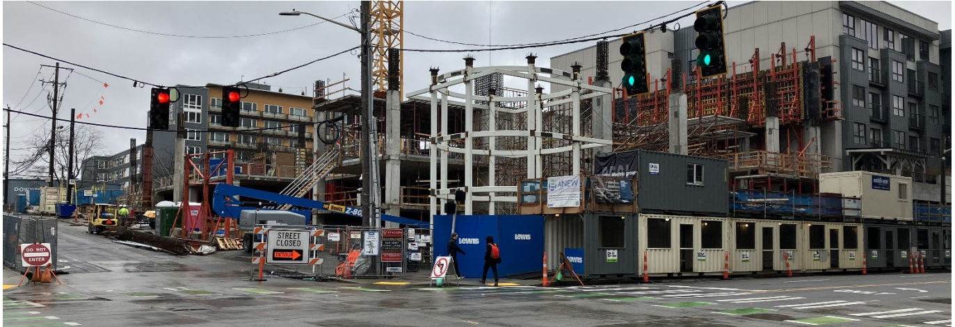
Construction Progress at 701 Dexter (February 2023)
