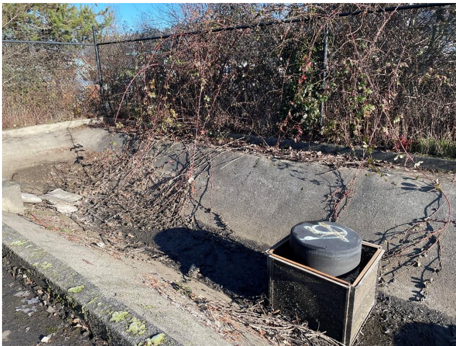
Photo 16 (facing north): View of a treatment basin on the northern portion of the Site. Some sediment and vegetation are visible.
