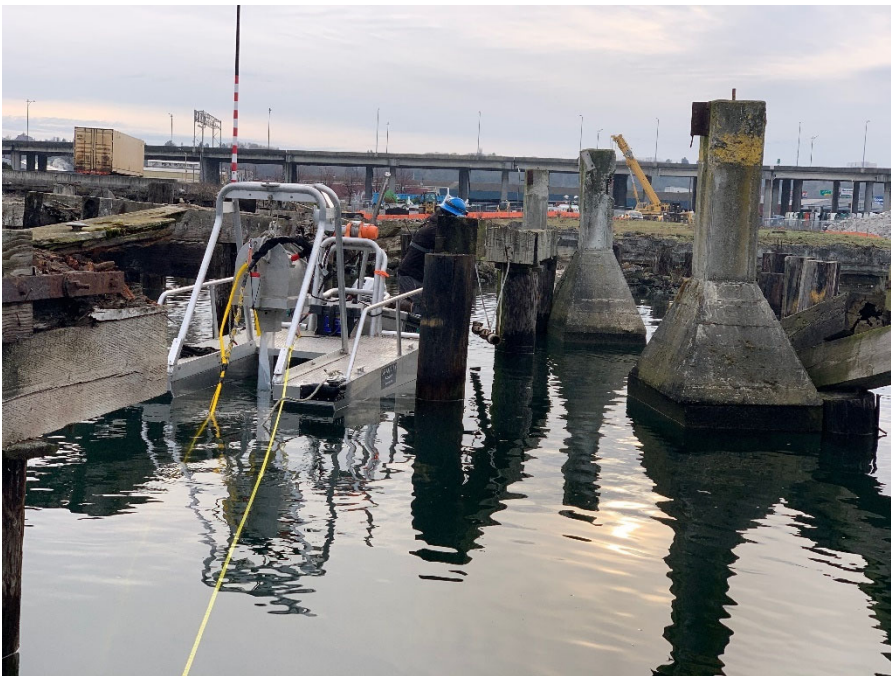
Float Frame for Deployment in the Pile Field
