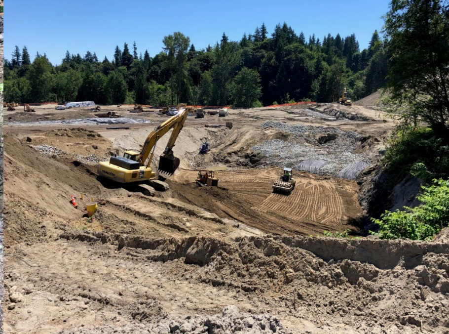
Excavation Landfill Material from Wedge Area
