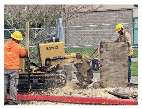
Photo 5. Contractor grinding the stumps.
