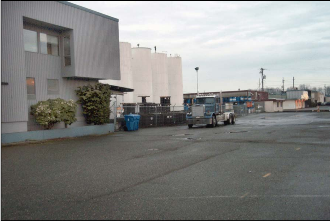
Figure 8. Overview of Pacific Functional Fluids complex, view to the northwest.
