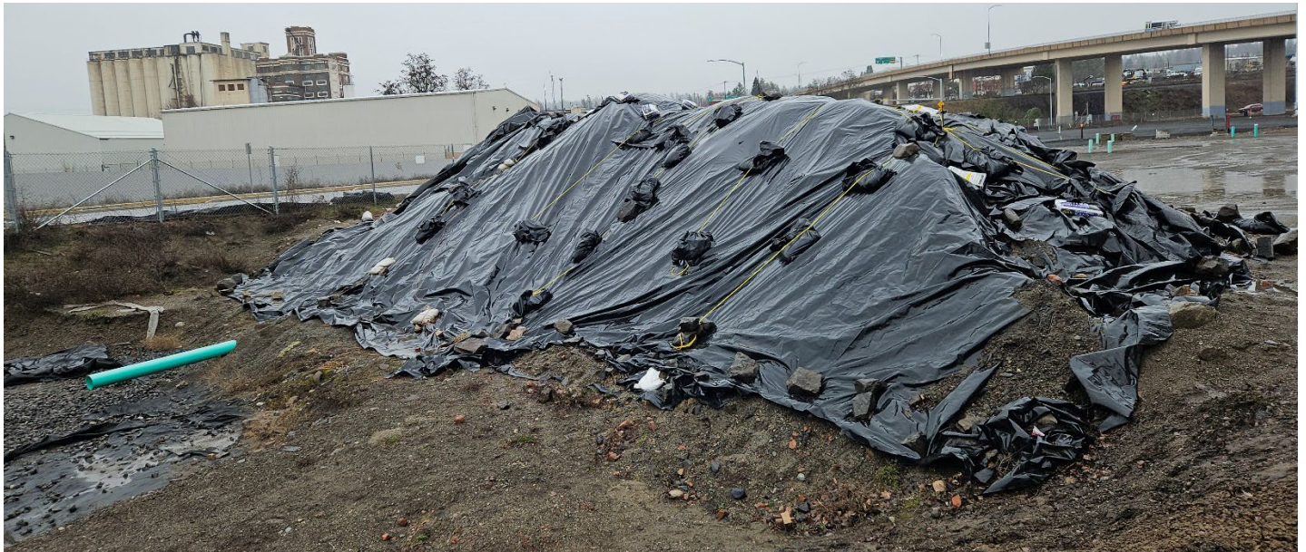
Photograph 8 – Soil stockpile cover
