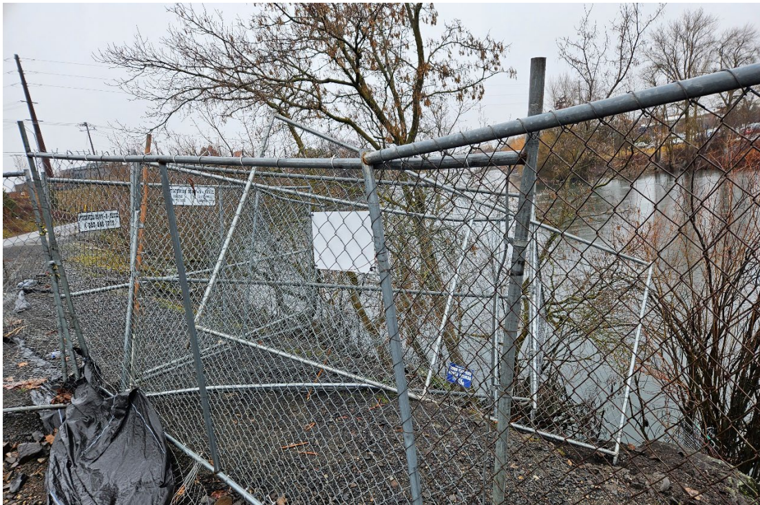
Photograph 2 – West extent of security fence
