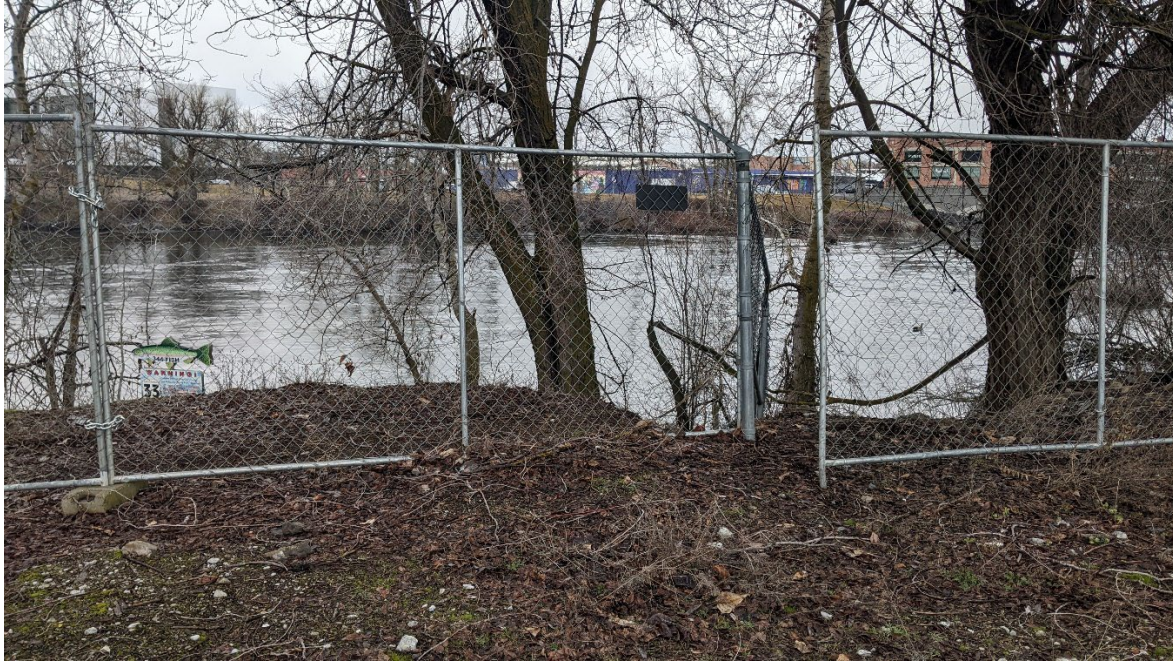
Photograph 1 – East extent of security fence
