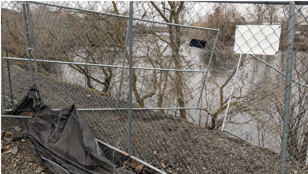
Photograph 2 – West extent of security fence
