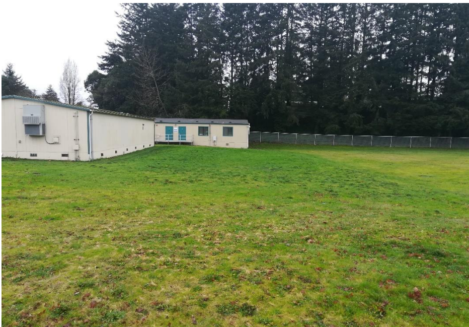
Photo Location 2. 12/16/2020 site inspection
