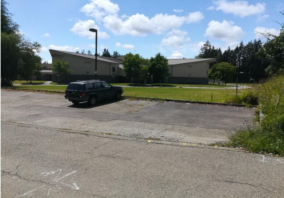
Photo Location 1. 6/11/2020 site inspection
