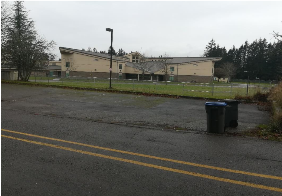
Photo Location 1. 12/16/2020 site inspection
