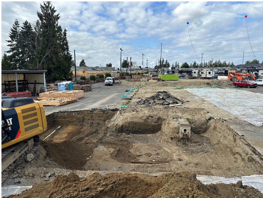
Photo 2. Remedial excavation as seen looking northwest on September 24, 2023. Oil Water separator visible in right center of frame.
