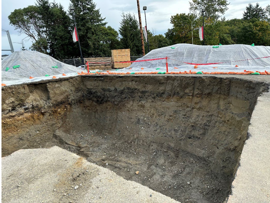
Photo 3. Remedial excavation as seen looking southeast on September 26, 2023. Clean overburden pile covered by white plastic visible top right of frame. A portion of the petroleum contaminated soil pile covered by white plastic is also visible top left of frame.
