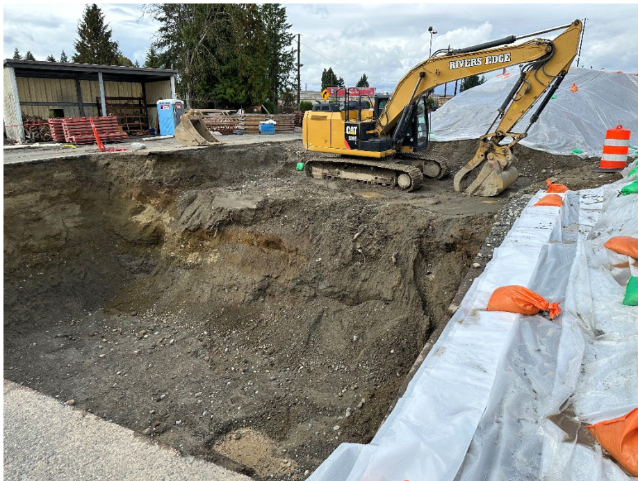
Photo 4. Remedial excavation as seen looking northwest on September 26, 2023.
