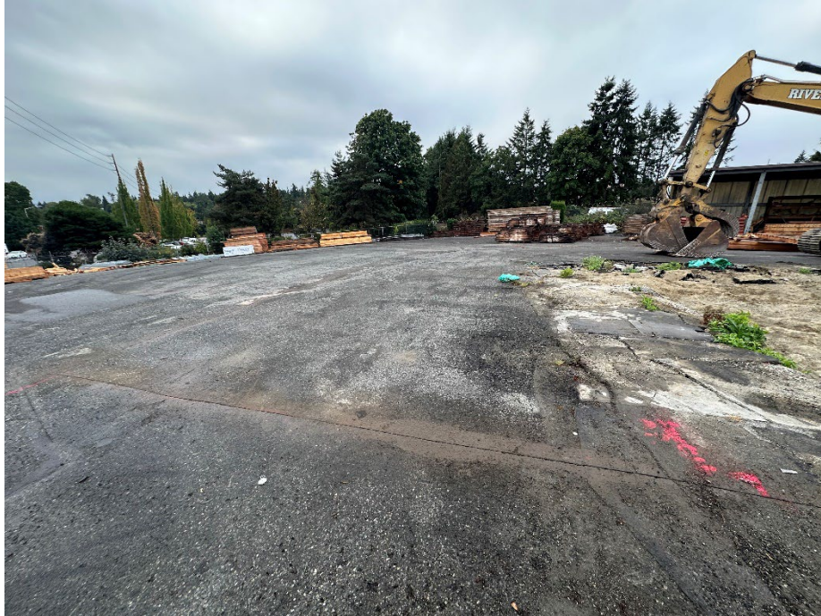
Photo 1. Excavation area as seen looking south on September 24, 2023.
