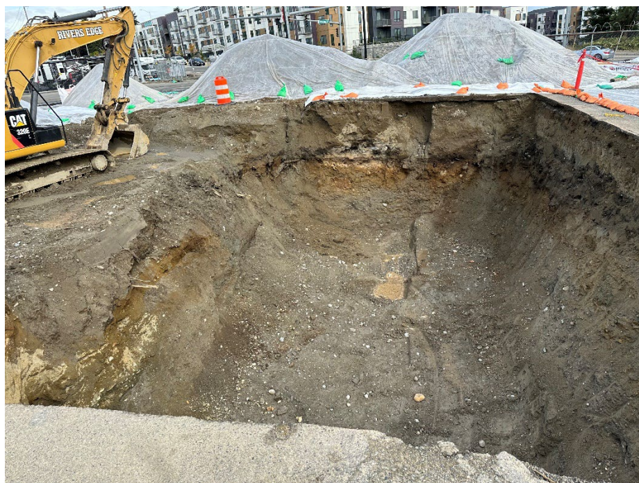
Photo 5. Remedial excavation as seen looking northeast on September 26, 2023.
