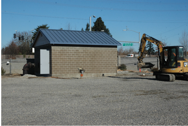
Photograph 1. Exterior view of well house.
