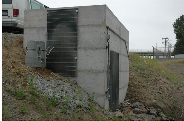
Photograph 9. Storm drain connection junction.
