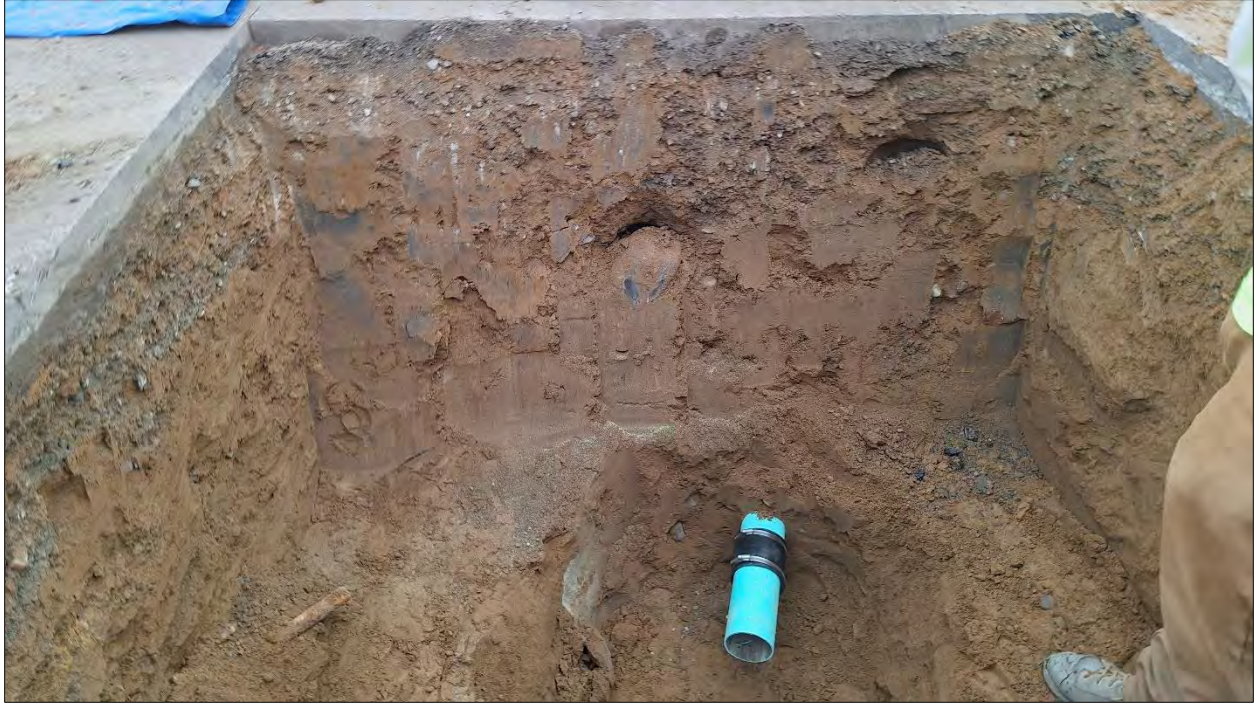
Figure 9. Overview of the excavated pit.
