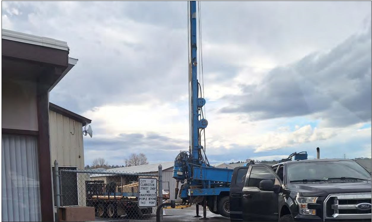
Figure 7. Overview of drilling activities. View to the south.
