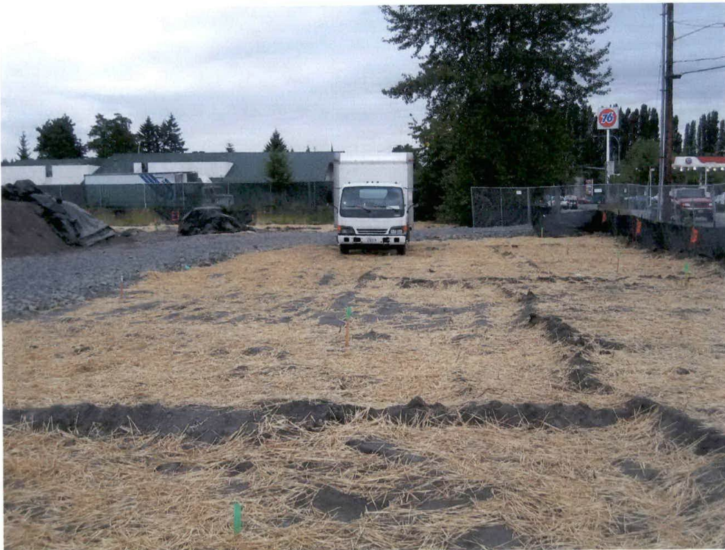
West to east view of completed excavation in southeast corner of site. Hay was spread over excavated area for erosion control.
