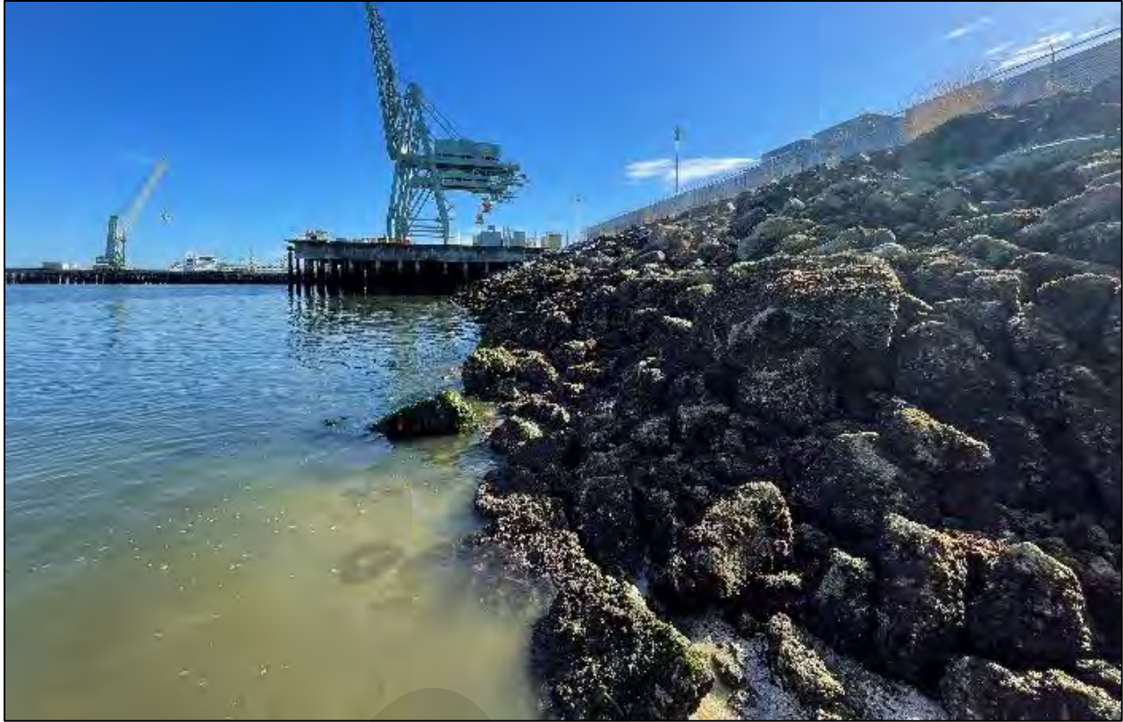
Photographs 1 & 2. Photo Point 1 in Area 1 of the Northern shoreline facing northeast (above) towards the Pacific Terminal, and southwest (below) towards the South Terminal; typical conditions. (See Figure 3 for approximate location.)
