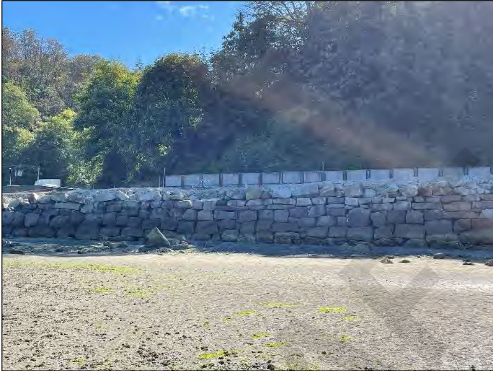
Photograph 36. Southern shoreline conditions near Pigeon Creek in Area B; typical. Vertical rock wall supporting the adjacent railroad tracks, facing South.
