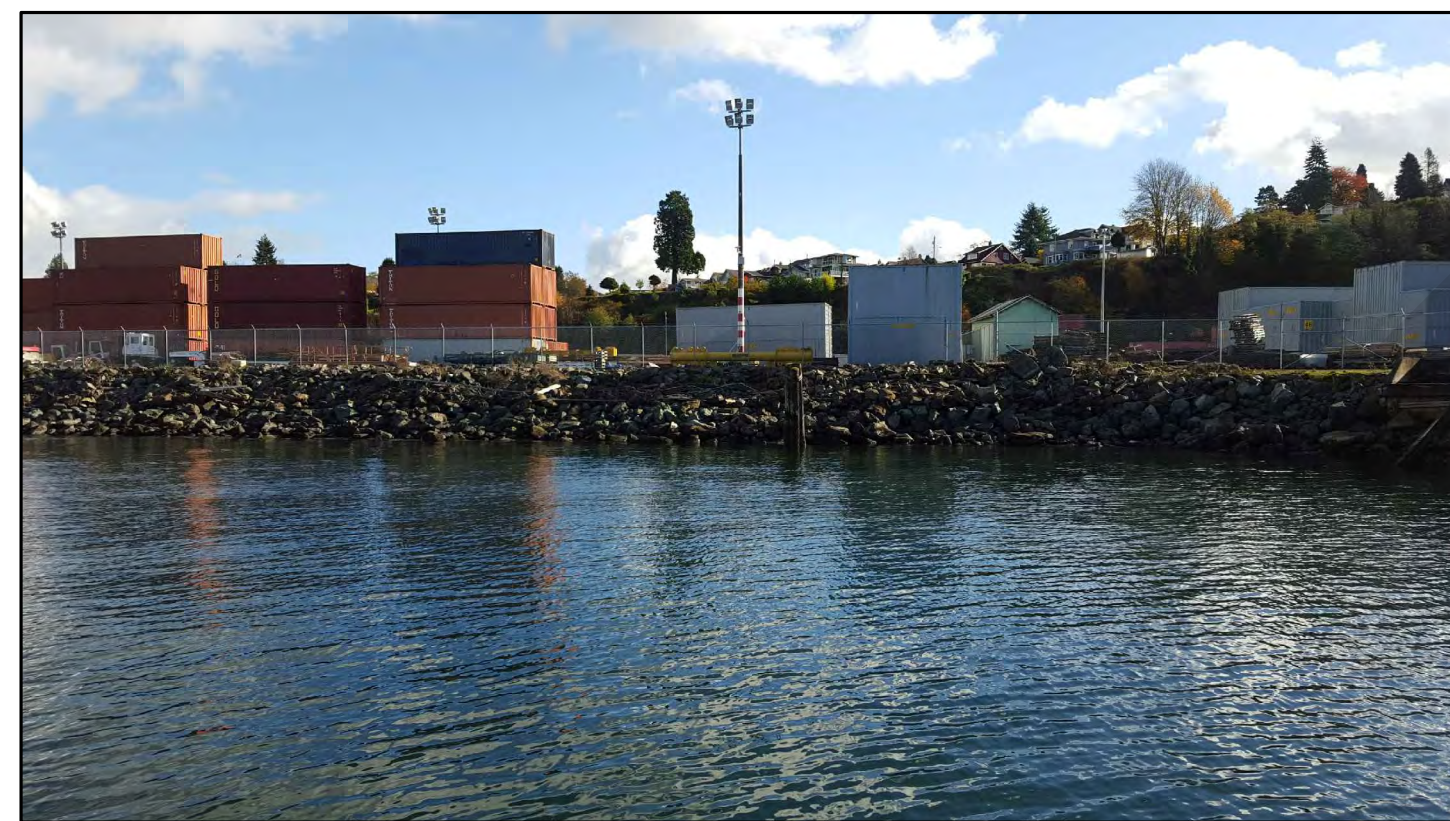
VIEW OF SOUTH TERMINAL SHORELINE LOOKING SOUTHEAST 4 3
