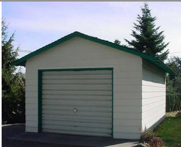
Photo 7: Sample Pb-7 White-Wood-Siding Lab data: 26,700 ppm
