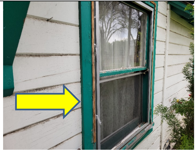
Photo 8: Sample Pb-8 Green-Wood-Window Casing Lab data: 29,100 ppm
