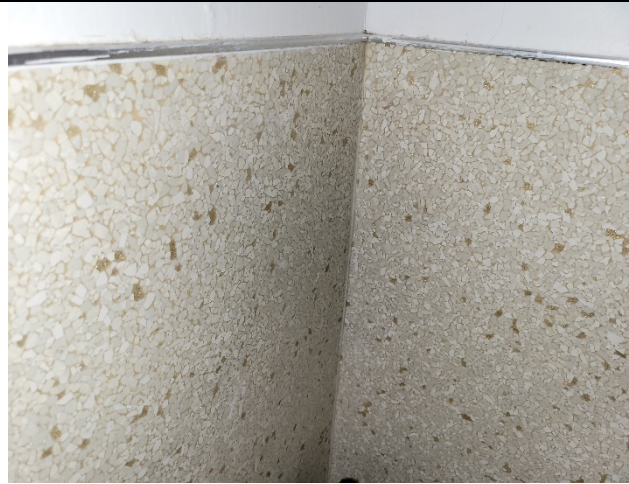
Photo 10: Sample #505 Lab data: Vinyl-Chrysotile-15% Mastic-Chrysotile-4%
