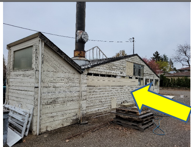
Photo 10: Sample Pb-10 White-Wood-Siding Lab data: 19,400 ppm
