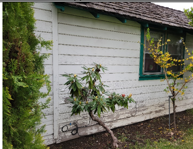
Photo 6: Sample Pb-6 White-Wood-Siding Lab data: 15,200 ppm
