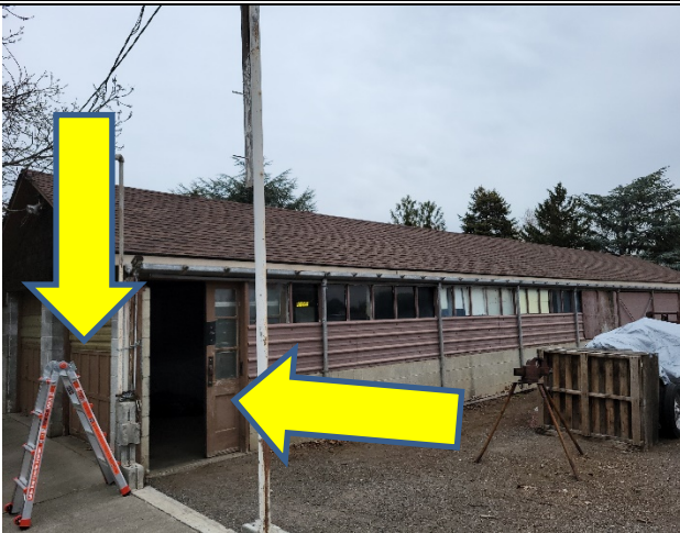
Photo 11: Sample Pb-11 Brown-Wood-Doors Lab data: 90,800 ppm
