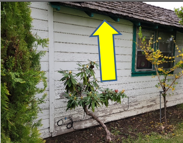
Photo 9: Sample Pb-9 Green-Wood-Soffit/Trim Lab data: 32,700 ppm
