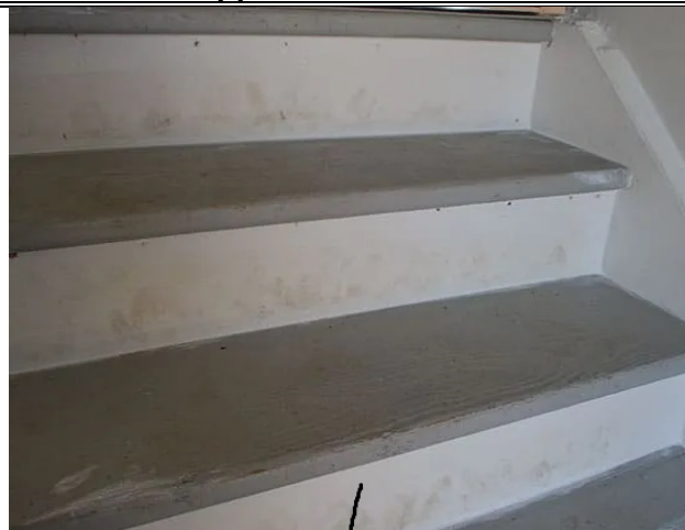
Photo 4: Sample Pb-4 Gray-Wood-Stairs Lab data: 25,000 ppm
