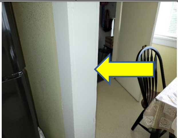
Photo 3: Sample Pb-3 White-Wood-Door Casing Lab data: 1,590 ppm
