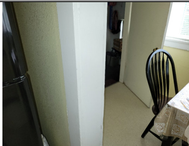
Photo 2: Sample Pb-2 Yellow-Gypsum Wallboard-Walls Lab data: 705ppm
