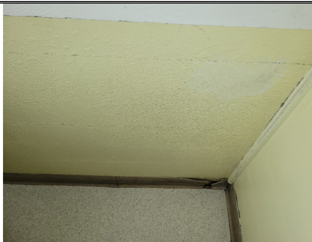
Photo 1: Sample Pb-1 Yellow-Wood-Wainscot Lab data: Below Reportable Limit
