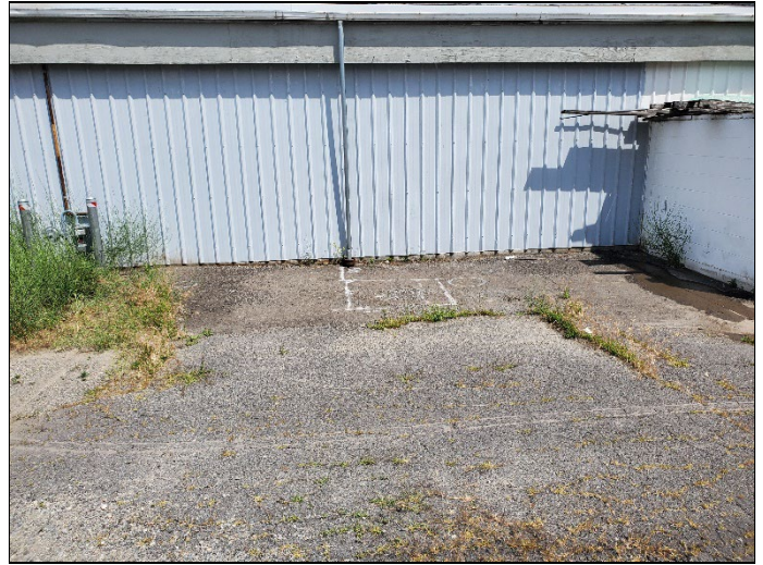
2. Drywell location as marked previously in March 2023 LESE ground penetrating radar locate
