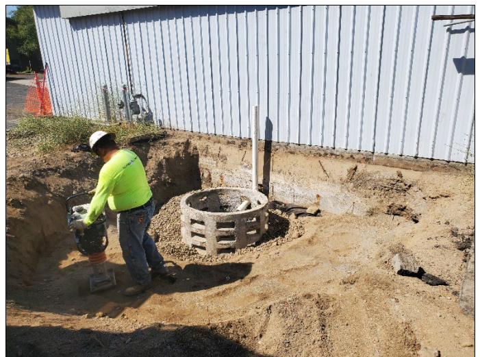
6. Replacement of drywell, roof-drain connection, drainrock, and surrounding soil
