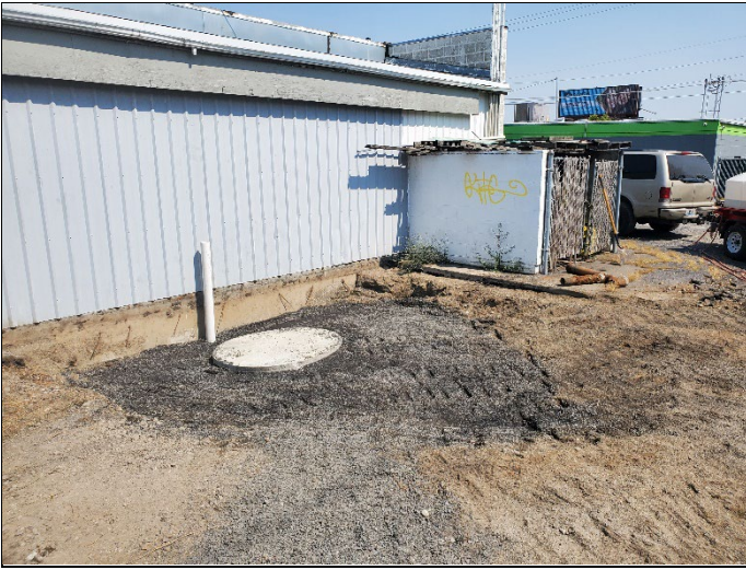
7. Replaced lid over drywell
