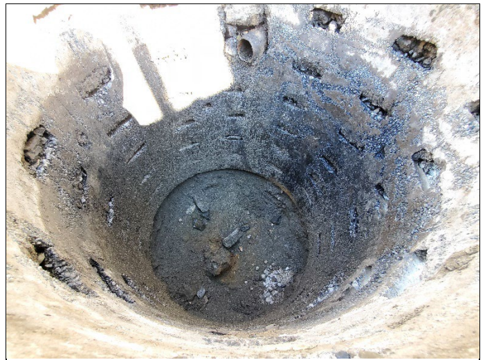
4. Drywell after vac-truck
