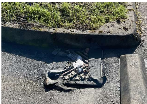
SW-3 - Catch basin still has obstructions though less than during previous inspection
