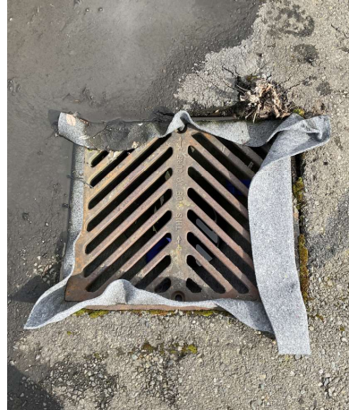
SW-3 - Catch basin still has obstructions though less than during previous inspection
