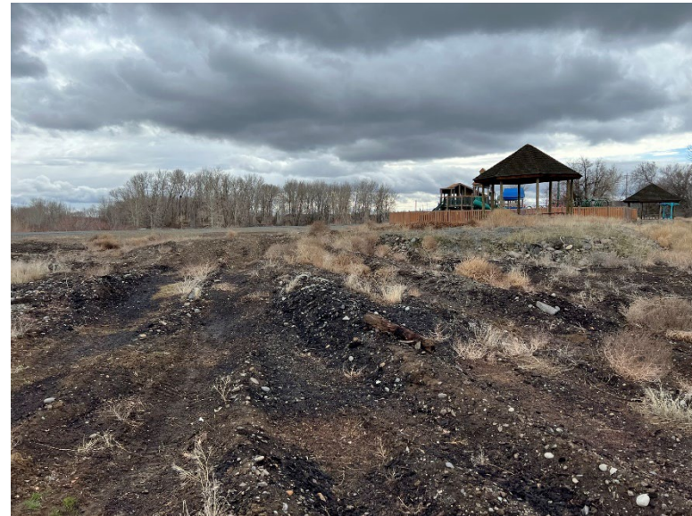
B24.4 Parcel E – Log yard material is present near the playground.
