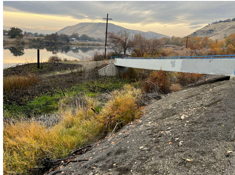
B2.4 Parcel A – Bridge connecting Yakima Greenway to Rotary Lake.
