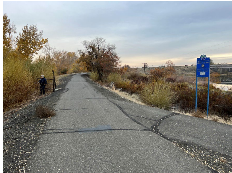
B3.4 Parcel A – Looking south from near the head gate at Parcel A.
