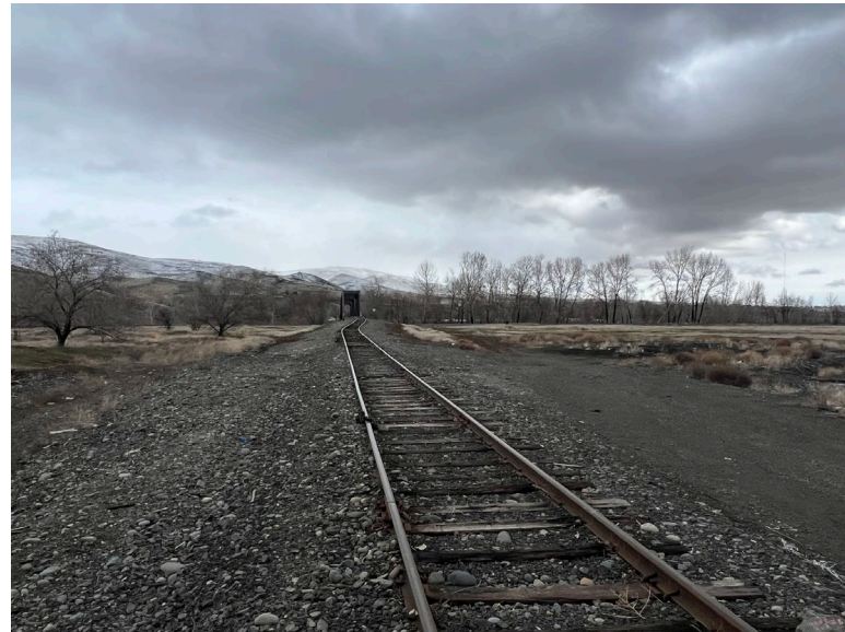
B17.4 Parcel D – The railroad tracks looking east at the bridge over the Yakima River.
