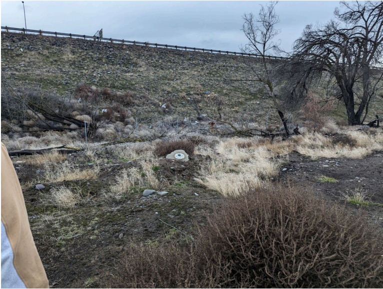
B26.1 Parcel E – A flush mount well monument located in the approximate future East-West Corridor roadway path.
