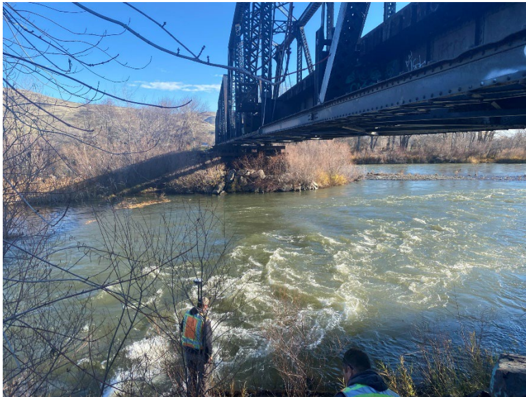
B19.1 Parcel D – The railroad bridge over the Yakima River.
