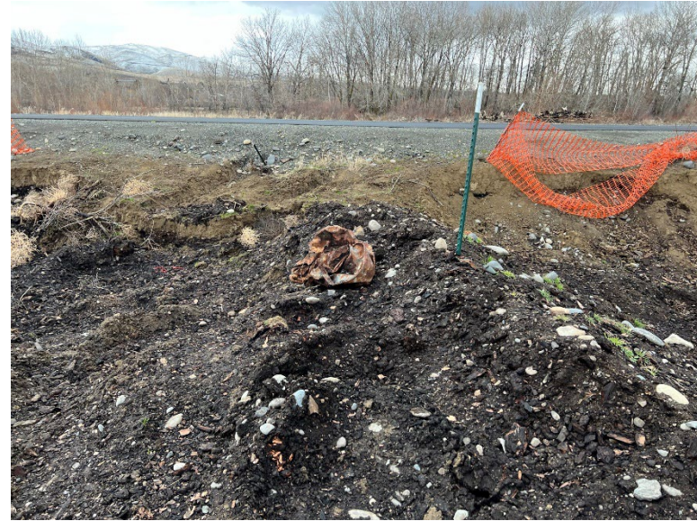
B24.2 Parcel E – Metal debris, including a crushed drum, was observed in the excavated area of log yard material.
