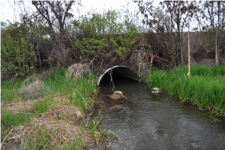
B20.1 – The Fruitvale Wasteway conveyance observed in April 2017.
