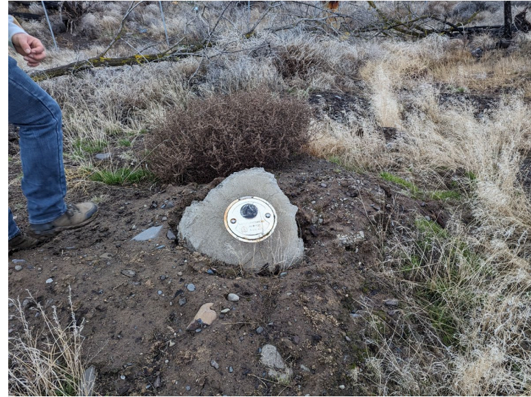
B26.2 Parcel E – The well monument appears to have been pulled from the ground.
