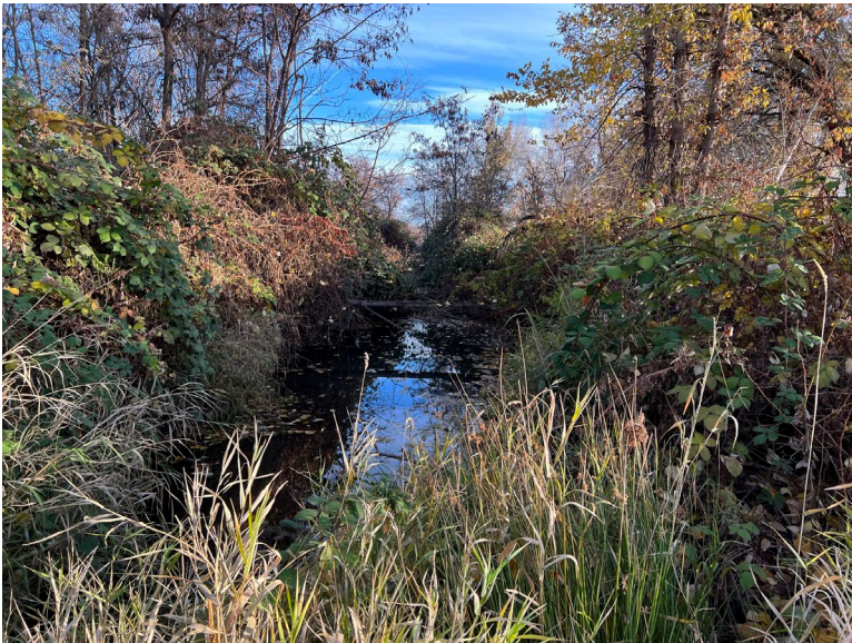
B15.3 Parcel D – The combined ditch is heavily vegetated.
