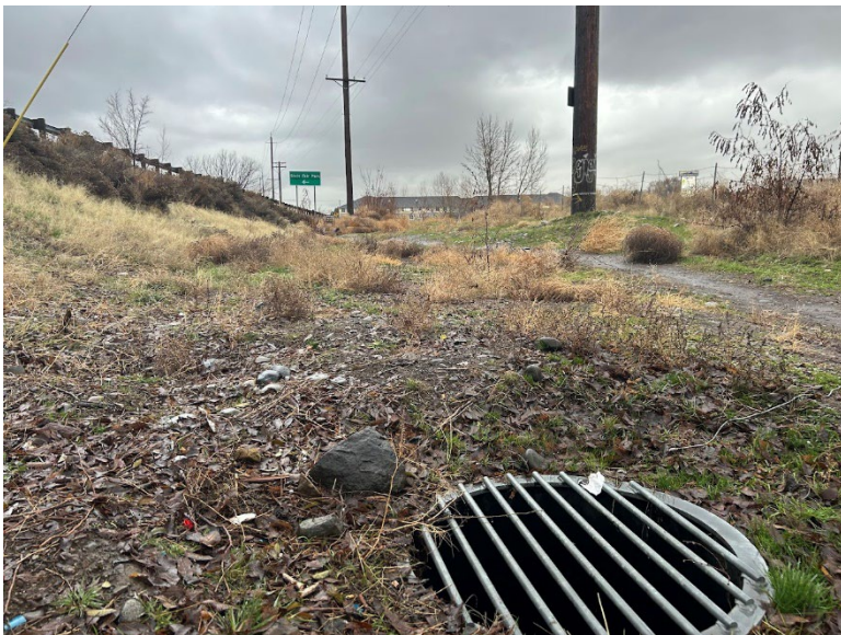
B20.3– The Fruitvale Wasteway is conveyed in piping along the south half of the Landfill Parcel.
