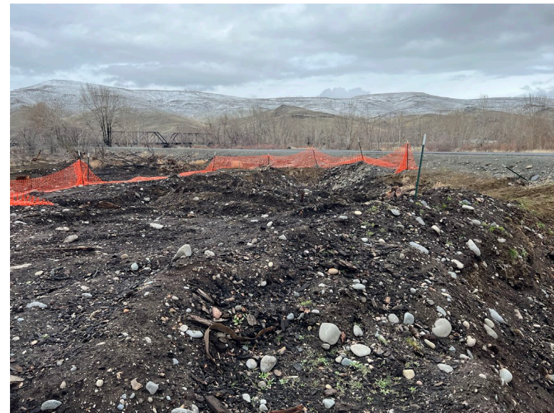
B18.4 Parcel E – The log yard material consists of mixed soil, wood debris, and rock.
