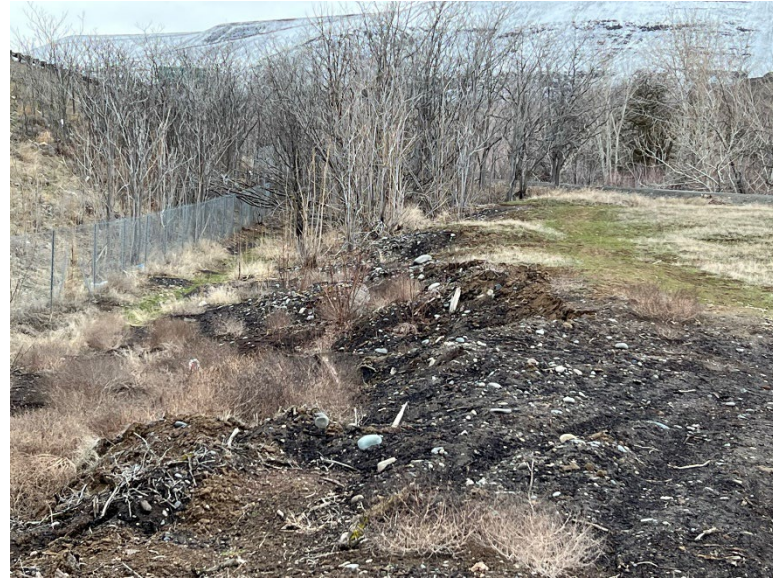
B25.2 Parcel D – Log yard materials are present at the ground surface and the elevation changes about 6-feet to the fence.
