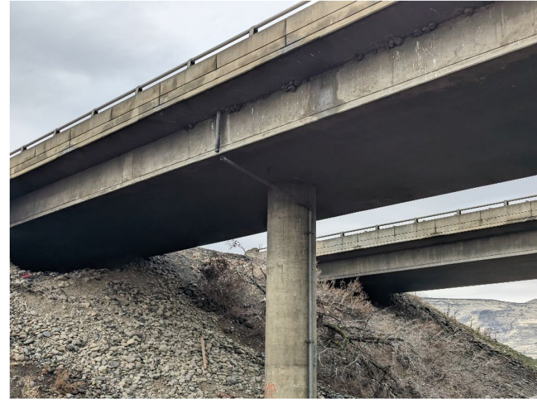
B21.2 Parcel E – A connective elbow is missing on the downspouts. Water discharges to the ground surface.
