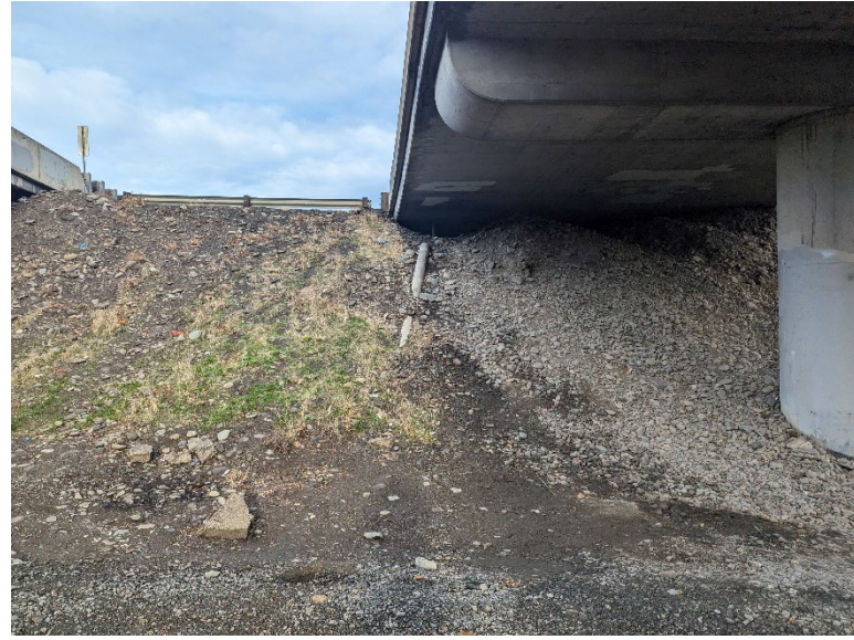
B23.2 – One of the metal culverts present beneath the overpass.
