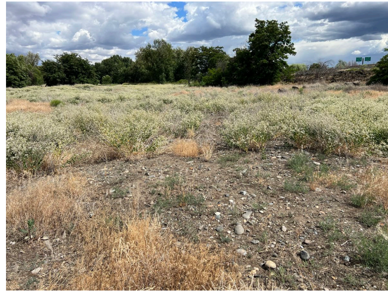
B8.2 Parcel C1 – The area east of the parking lot is the former interstate borrow pit footprint.
