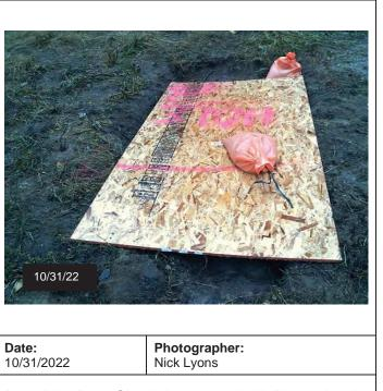
Demolition Prep, Shot holes covered with Plywood and marked "HOLE"
