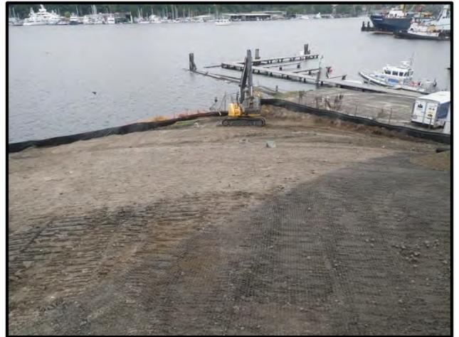
We also observed the contractor preparing the subgrades for the paved pedestrian paths on the north side of Kite Hill. The contractor placed approximately 6-inches of Type 17 along the path alignment and compacted it with an Ingersoll Rand steel drum vibratory roller. After the Type 17 was compacted, we observed the contractor begin placing 5/8-inch minus crushed rock base course over it.
