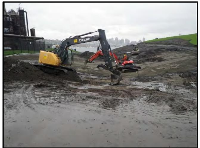
We also observed the contractor fine grading the path subgrade on the west side of the Cracking Tower and south west of the benches on the south side of Kite Hill (see attached site plan). The contractor was spreading 5/8-inch and/or 1 1/4-inch minus crushed rock base material in thin lifts and compacting it with a vibratory plate compactor and/or a Wacker RD12 dual drum articulated mini compactor.
