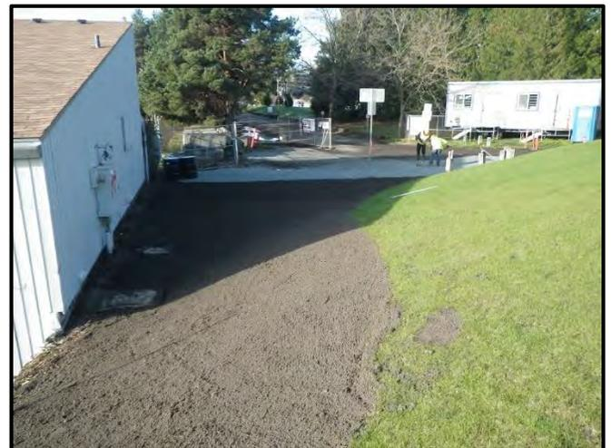
We also observed the contractor restoring the surfacing at the end of Northlake Way. The contractor placed and compacted an approximately 4-inch lift of 1 1/4-inch minus crushed rock base course. The crushed rock was compacted with a mini dual drum vibratory roller.
