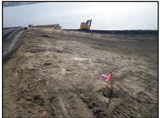
We also observed the contractor preparing the subgrades for the paved pedestrian paths on the south side of Kite Hill. The contractor placed approximately 6-inches of Type 17 at the path alignment and compacted it with an Ingersoll Rand steel drum vibratory roller. After the Type 17 was compacted, we observed the contractor begin placing 5/8-inch minus crushed rock base course over it.
