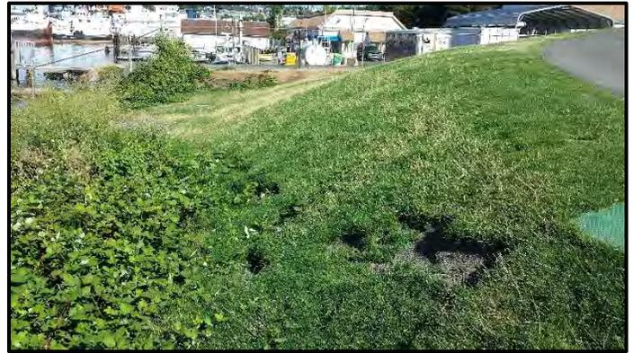
**Photo 3 - Loose sod along south side of Kite Hill**
