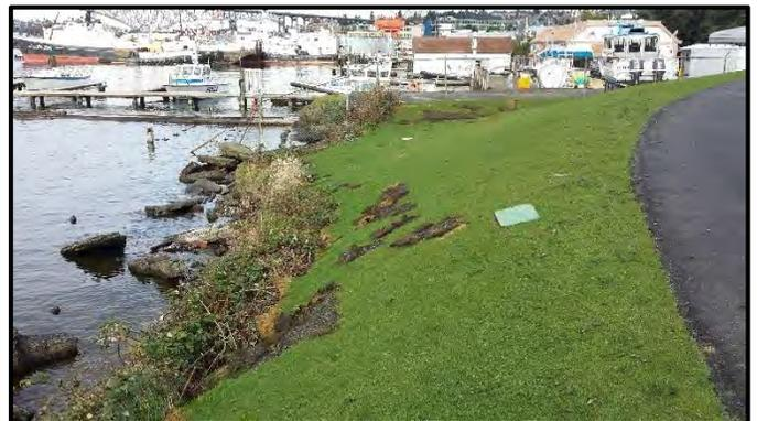
**Photo 5 - Areas of loose sod on south side of Kite Hill**
