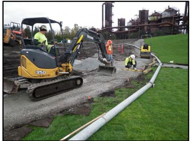
We also observed the contractor fine grading the path subgrade south west of the benches and on the south side of Kite Hill (see attached site plan). The contractor was spreading 5/8-inch and/or 1 1/4-inch minus crushed rock base material in thin lifts and compacting it with a vibratory plate compactor and/or a Wacker RD12 dual drum articulated mini compactor.
