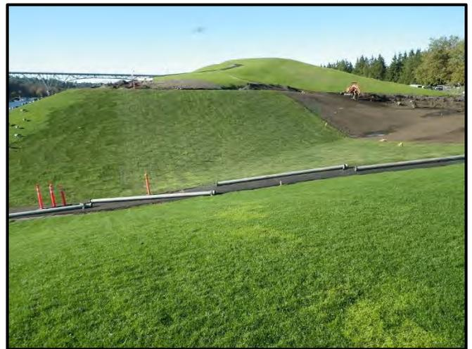
We also observed the contractor performing some fine grading of the topsoil in the swale area east of Kite Hill utilizing a Kubota track mounted mini excavator. The graded area was track compacted and/or tamped with the excavator bucket, and was being raked smooth by hand (see attached site plan).
