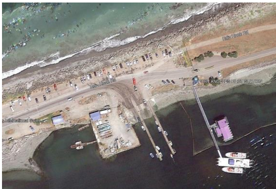
Figure 1. Former Cooke Aquaculture laydown area and associated derelict buildings.
